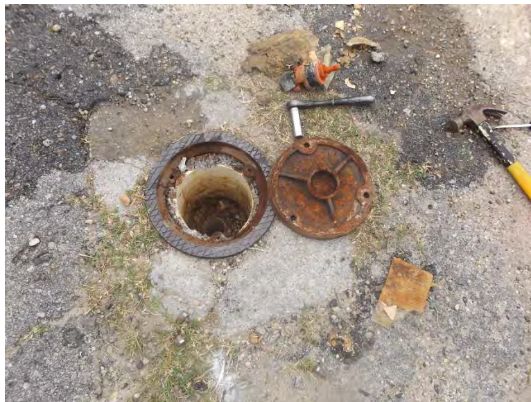
Photograph 5. Monitoring well DMW-1. Well depth measured at 45.4 feet. Depth to groundwater measured at 8.45 feet.
