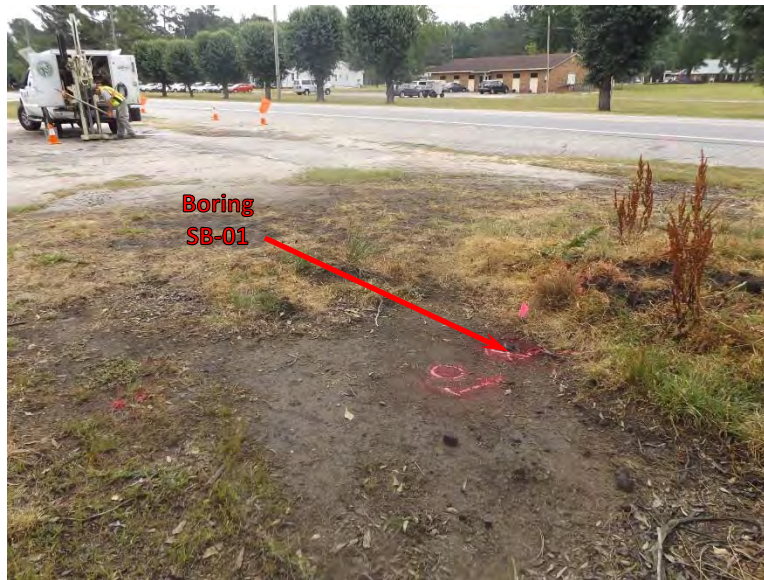
Photograph 6. GeoEnvironmental soil boring location SB-R5819-01.
