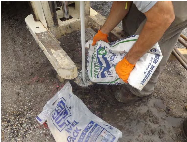
Photograph 11. Construction of temporary well GW-R5819-02 in GeoEnvironmental soil boring SB-R5819-02.
