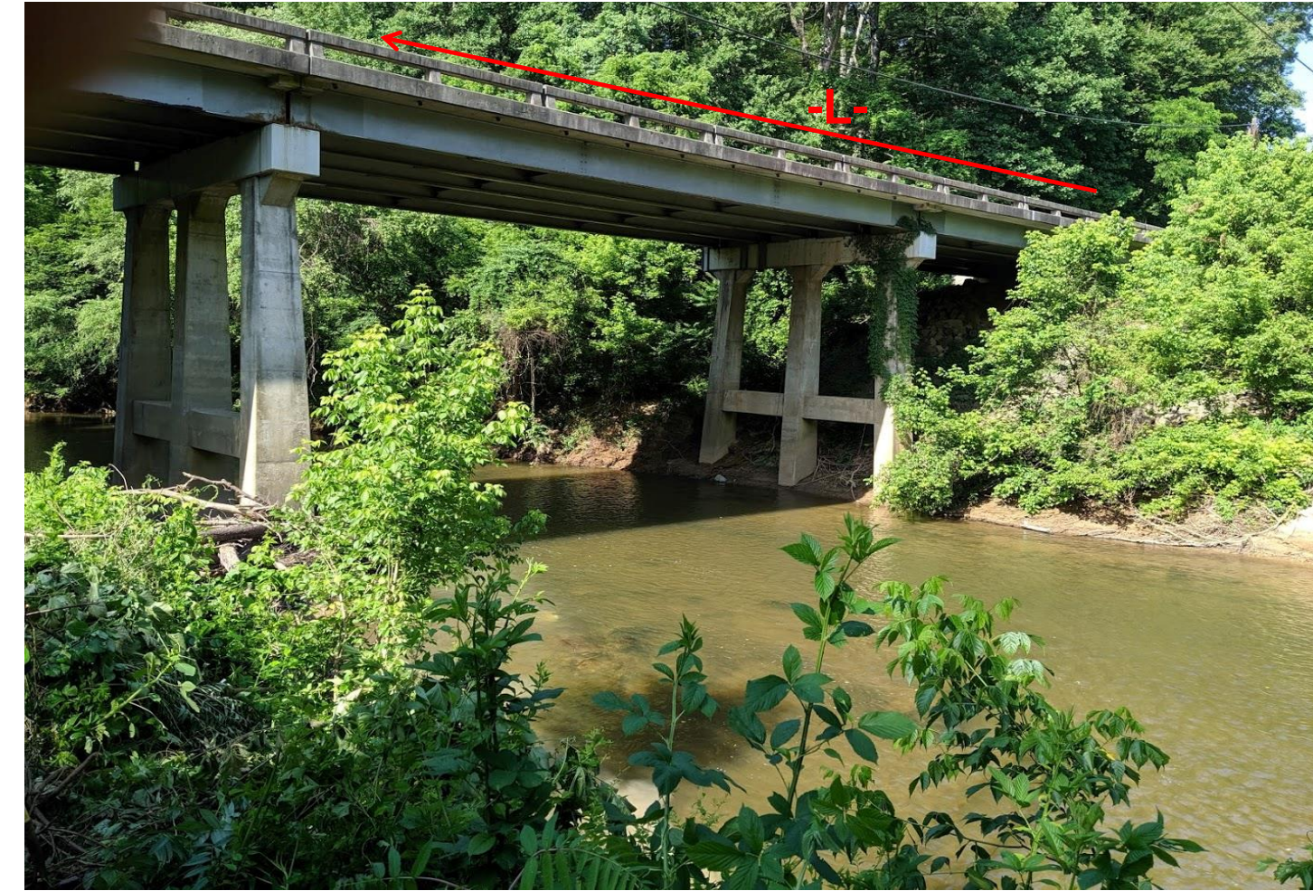
View from Downstream Side of Bridge
