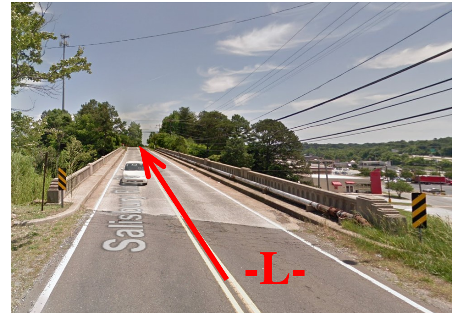
Standing at End Bent 1 Looking East toward End Bent 2
