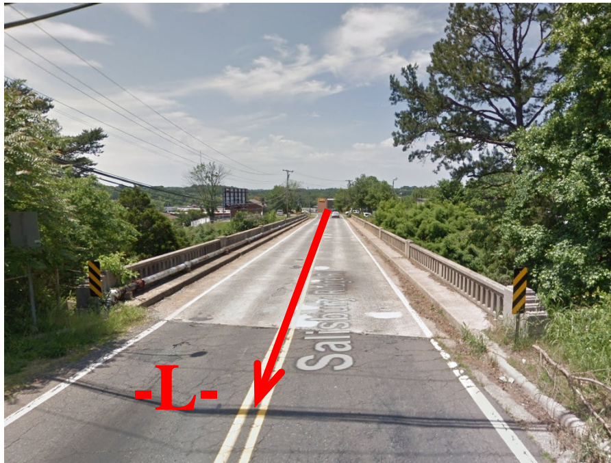
Standing at End Bent 2 looking west toward End Bent 1
