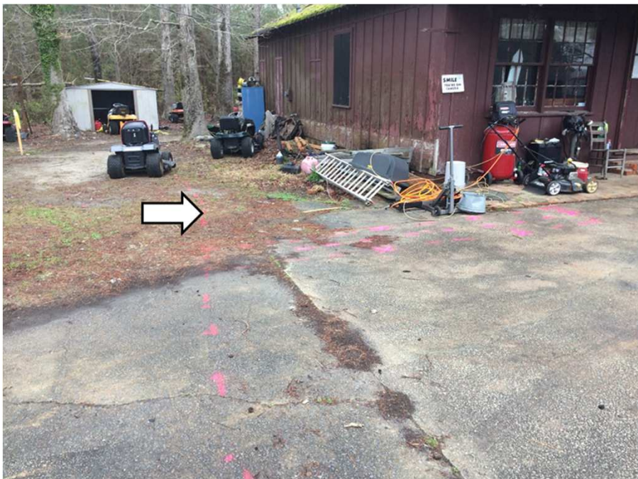
C. Possible area of former tank bed with line (arrow) traced from vent pipe on northeast corner of shop building.
