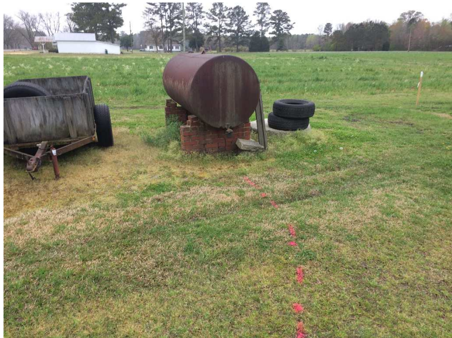
D. Approximate location of buried product line leading from AST to barn.
