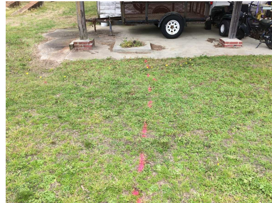
B. Possible relic product line leading west from pipe in middle of former dispenser pedestal, looking west.
