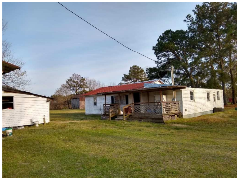
C. Photograph of second building on site and portion of survey area, looking southeast.
