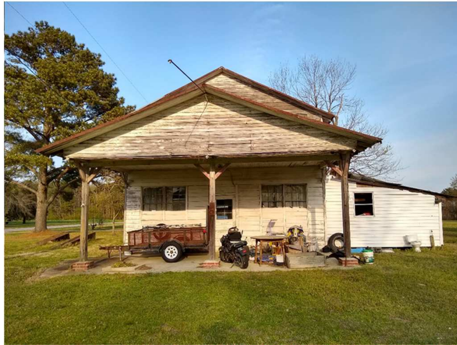
A. Front of former gas station building, looking east.
