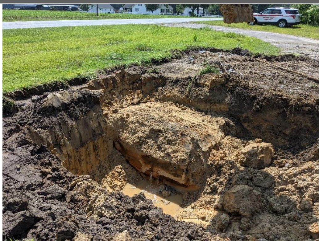
1 Description: Gas station USTs, uncovered
