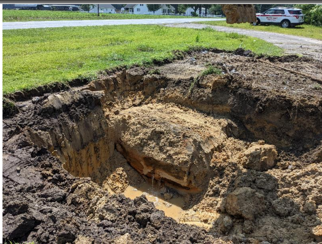
1 Description: Gas station USTs, uncovered
