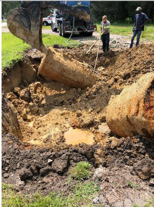
2 Description: Gas station USTs being removed
