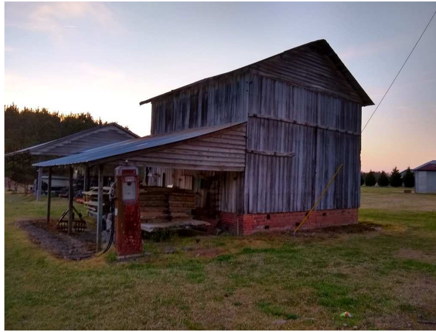
B. Photograph of barn number one showing the old UST pump and probable UST marked on the eastern corner, taken looking west.
