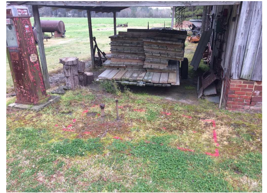
C. Close-up of probable UST marked on east side of barn number one (middle structure) on Parcel 137. Probable UST is approximately 3 feet diameter by 8 feet long.
