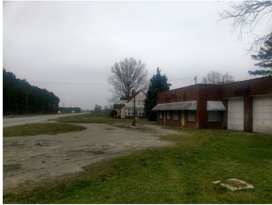
A. Photo from southwest side of site, looking northeast.
