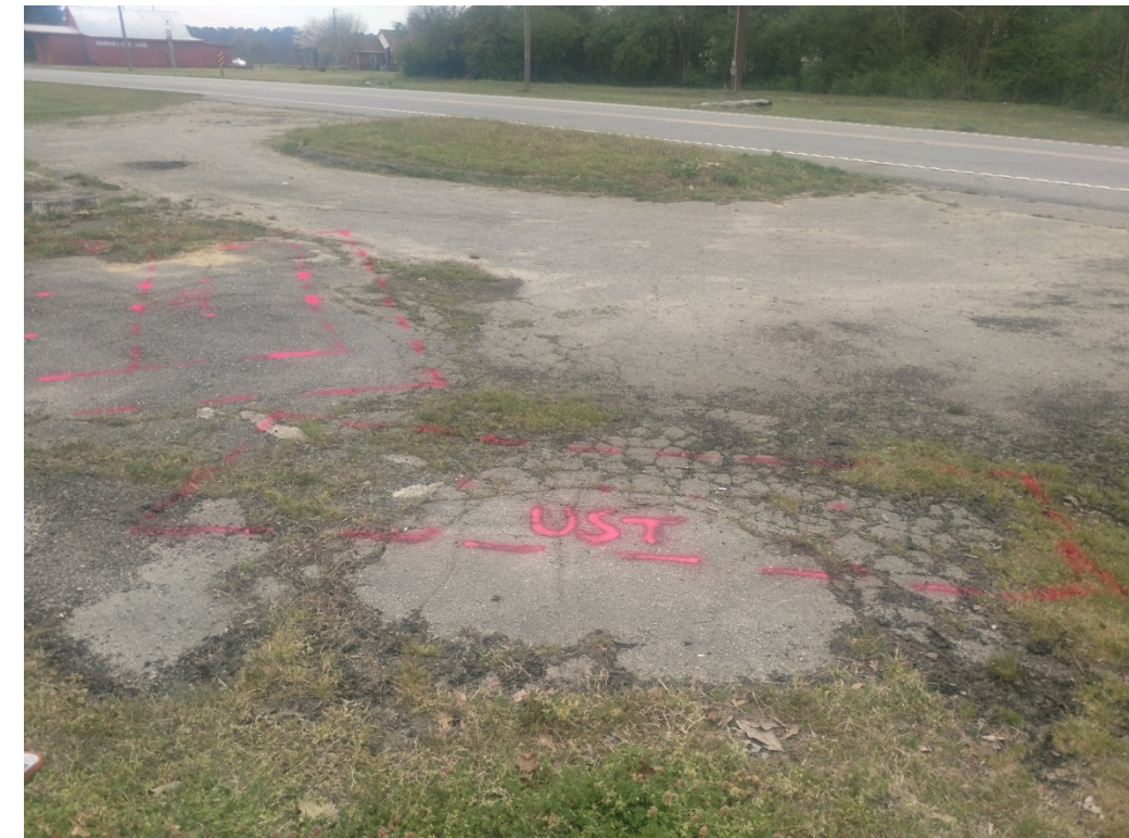
E. Photo of marked location of probable UST, looking west.
