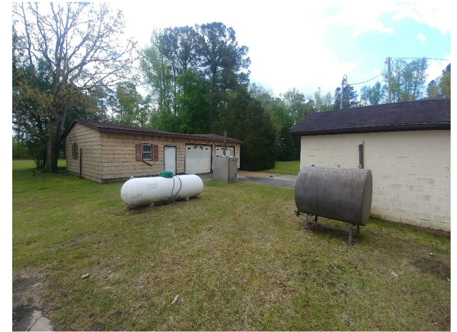
C. Photo of two ASTs behind residence.
