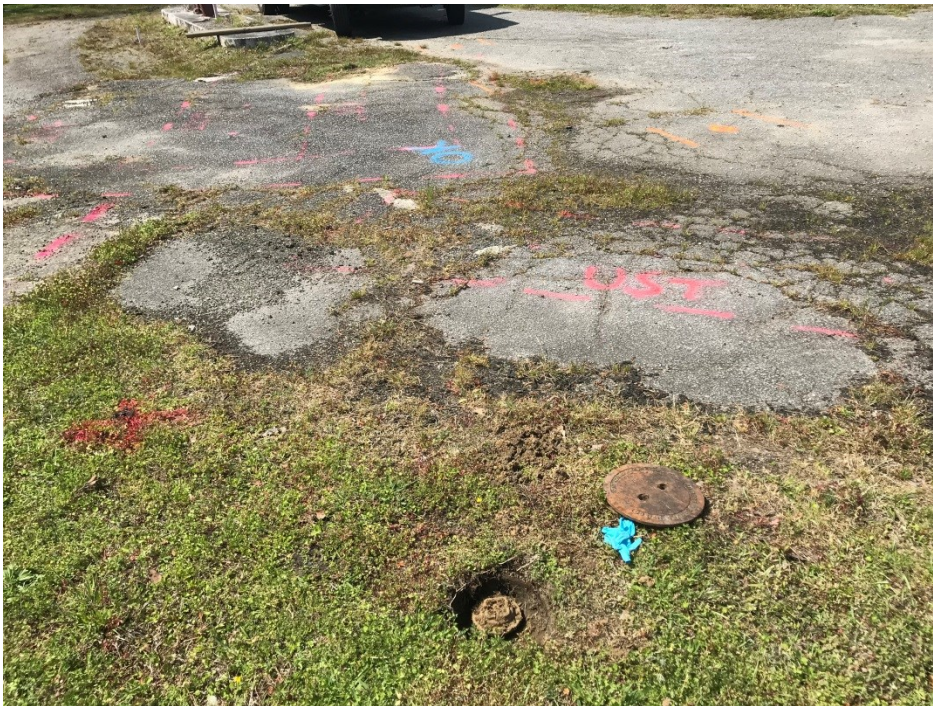
Photograph 6: View of UST basin and fill port.
