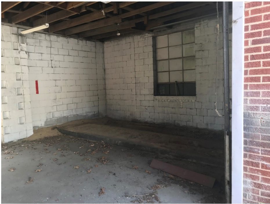
Photograph 3: View of the subject site interior – former automotive service facility.
