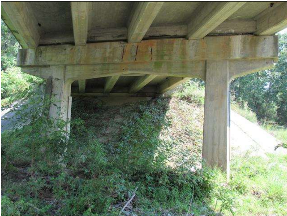
BENT 5, NEAR FACE
