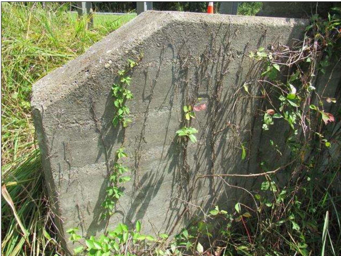
TYPICAL WINGWALL, FAR LEFT
