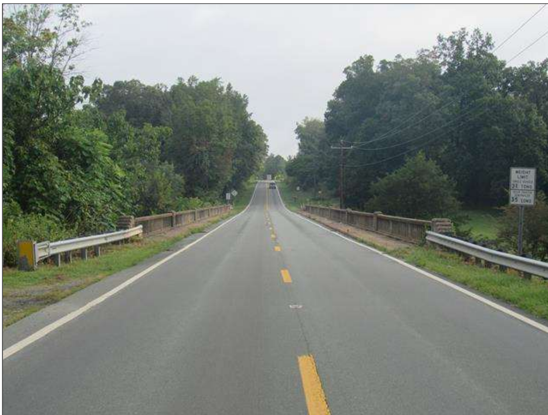
LOOKING STATIONS AHEAD, NORTH
