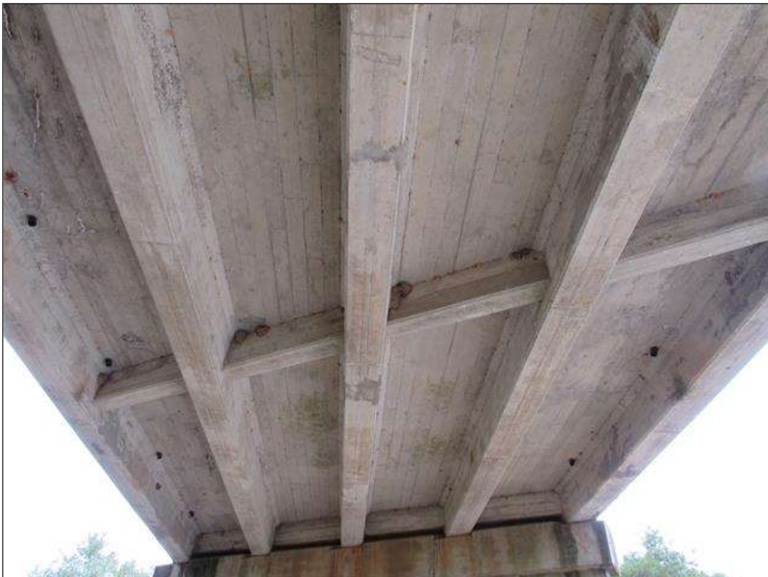
TYPICAL SUPERSTRUCTURE, SPAN 3 LOOKING AHEAD
