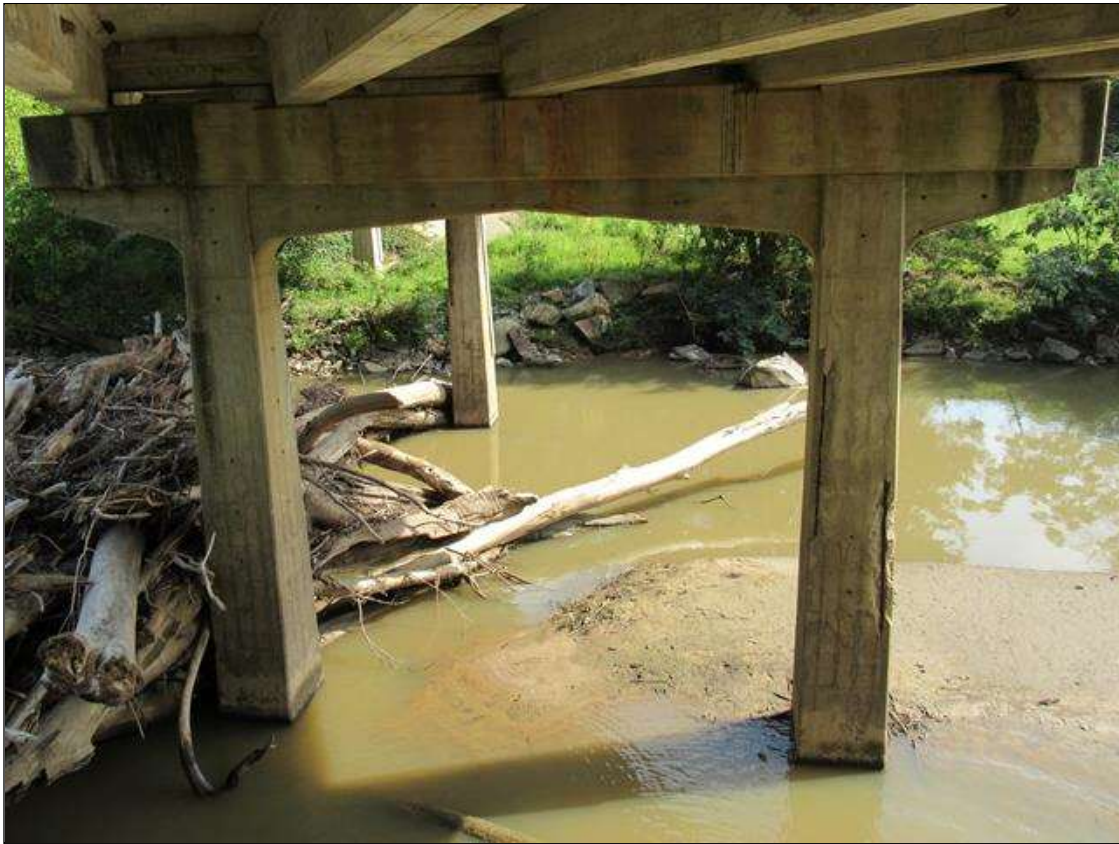
BENT 3, NEAR FACE
