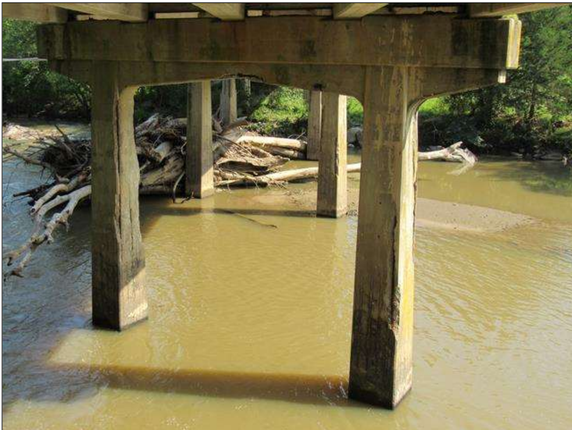
BENT 2, NEAR FACE
