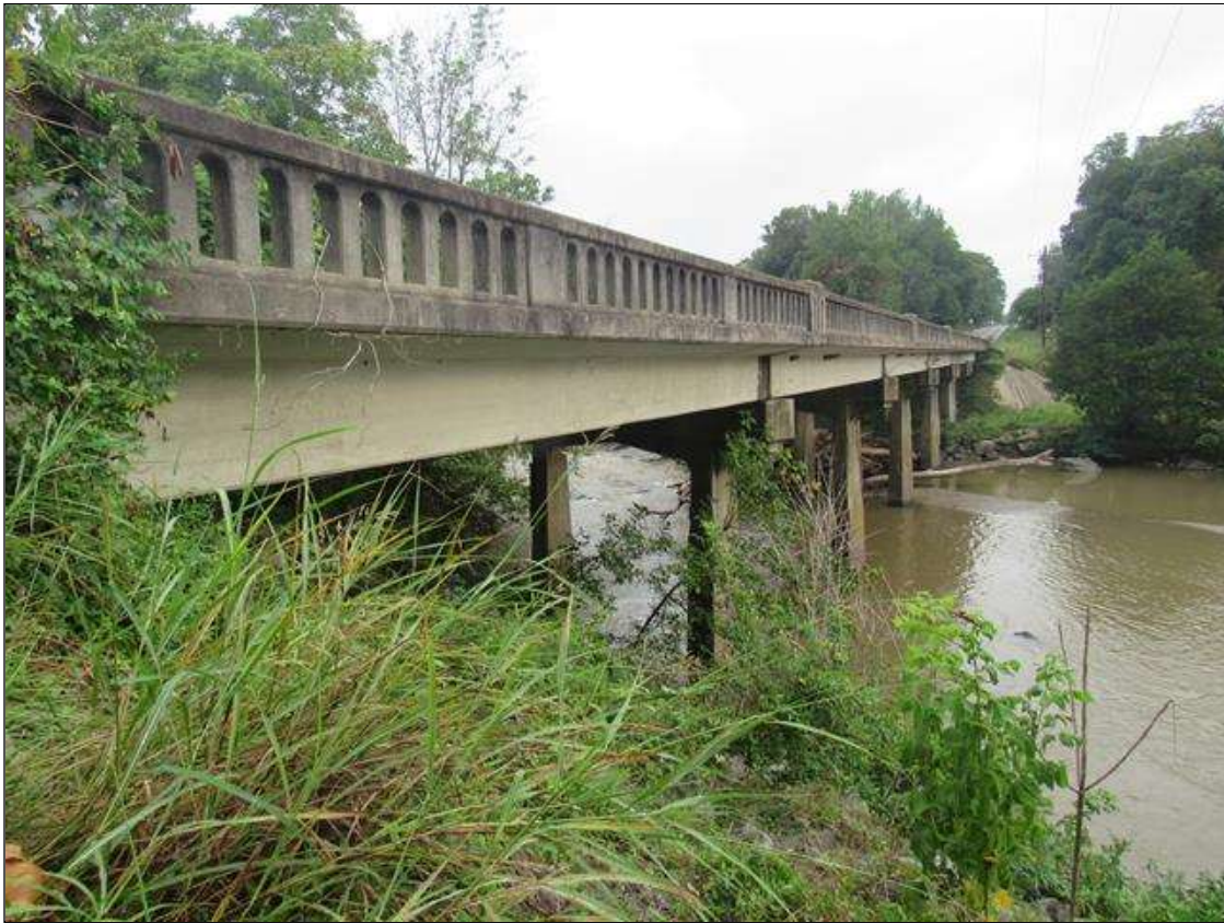
DOWNSTREAM ELEVATION, LOOKING AHEAD
