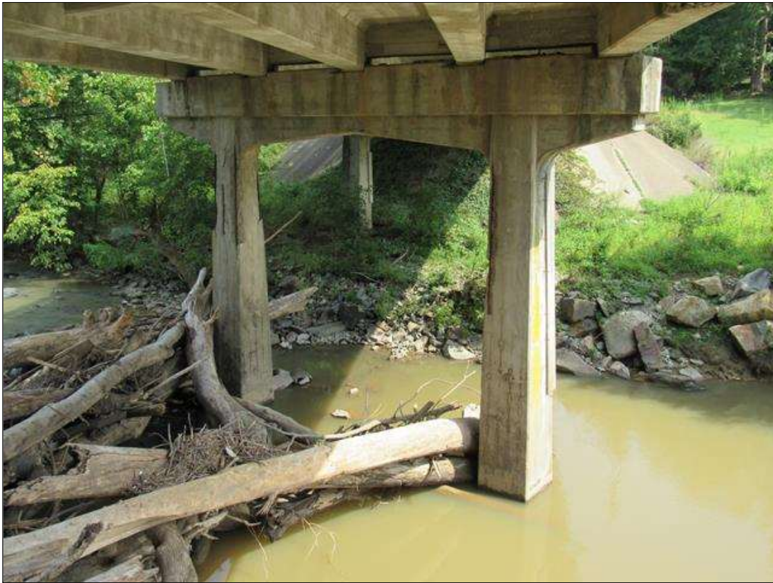
BENT 4, NEAR FACE
