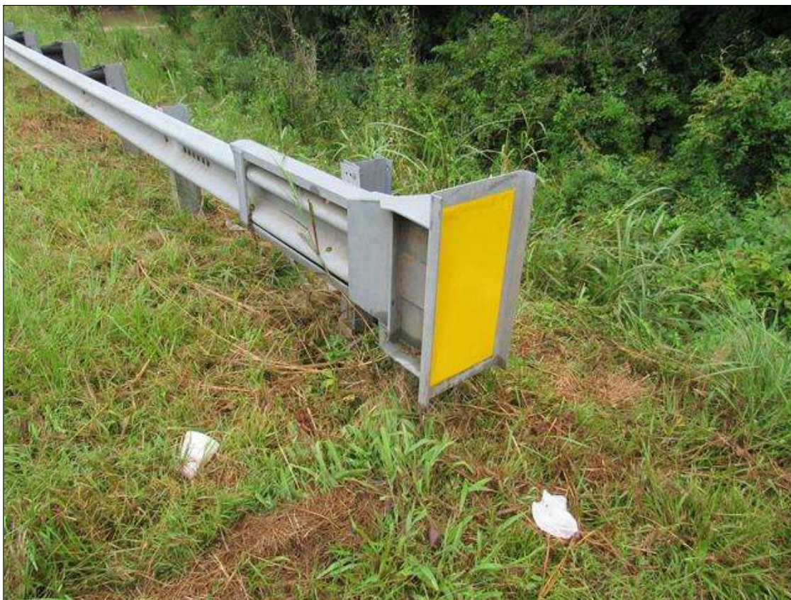
NEAR RIGHT GUARDRAIL END TREATMENT, NEAR LEFT SIMILAR
