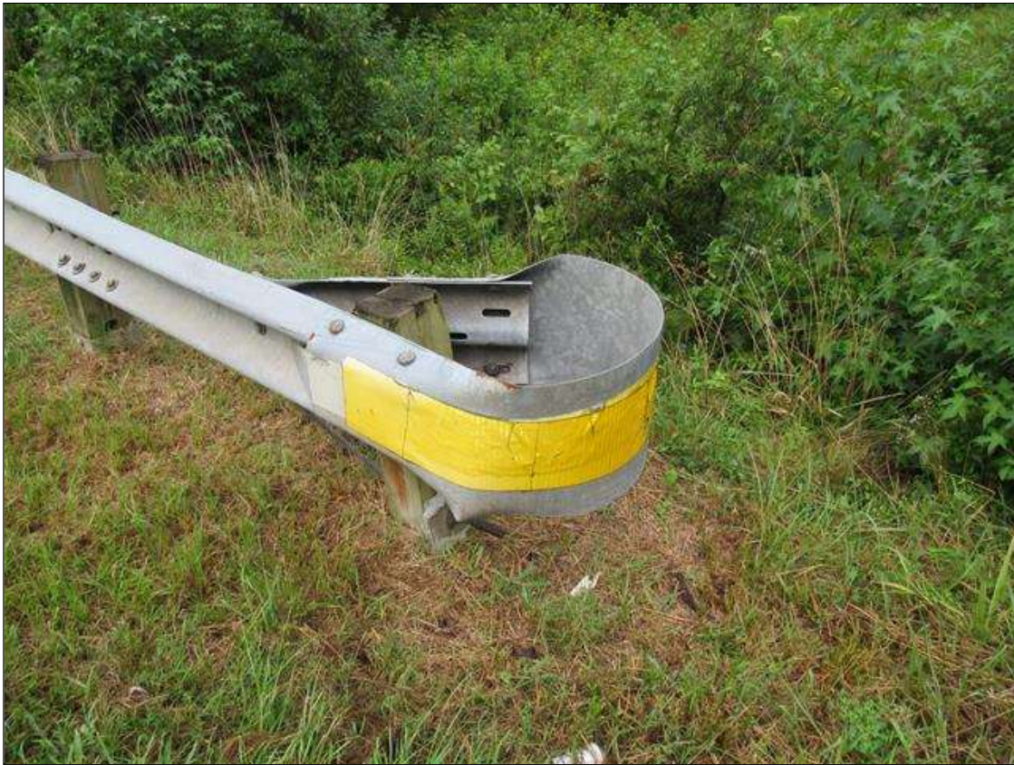
FAR LEFT GUARDRAIL END TREATMENT, FAR RIGHT SIMILAR
