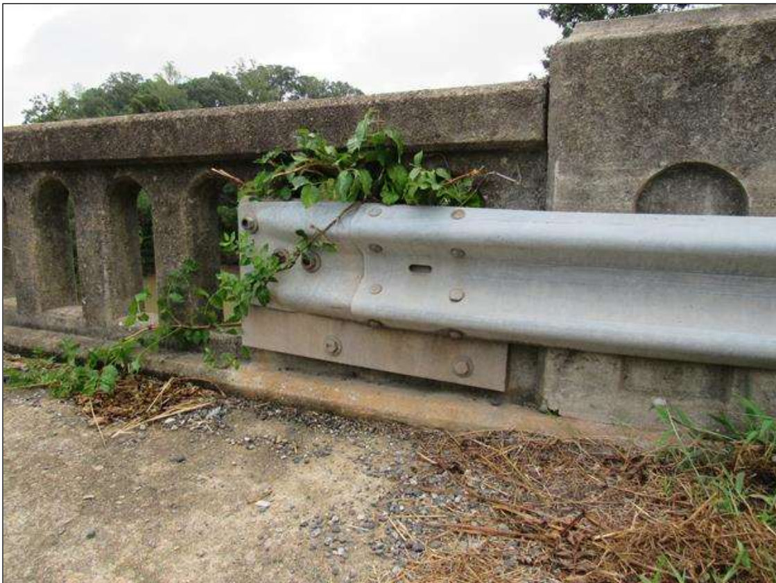
TYPICAL GUARDRAIL ATTACHMENT, NEAR RIGHT
