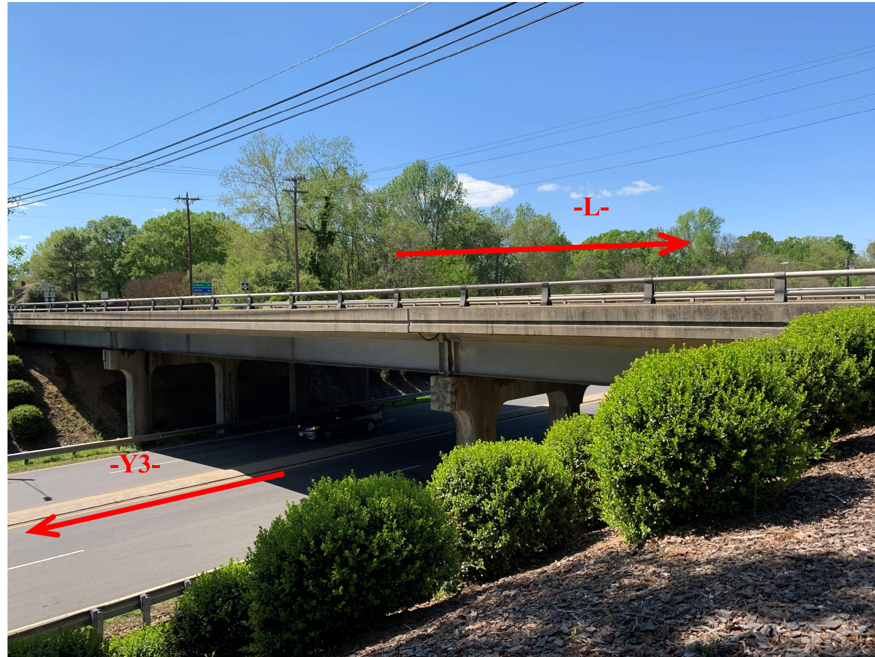
Looking Northwest at -L- from End Bent No. 2
