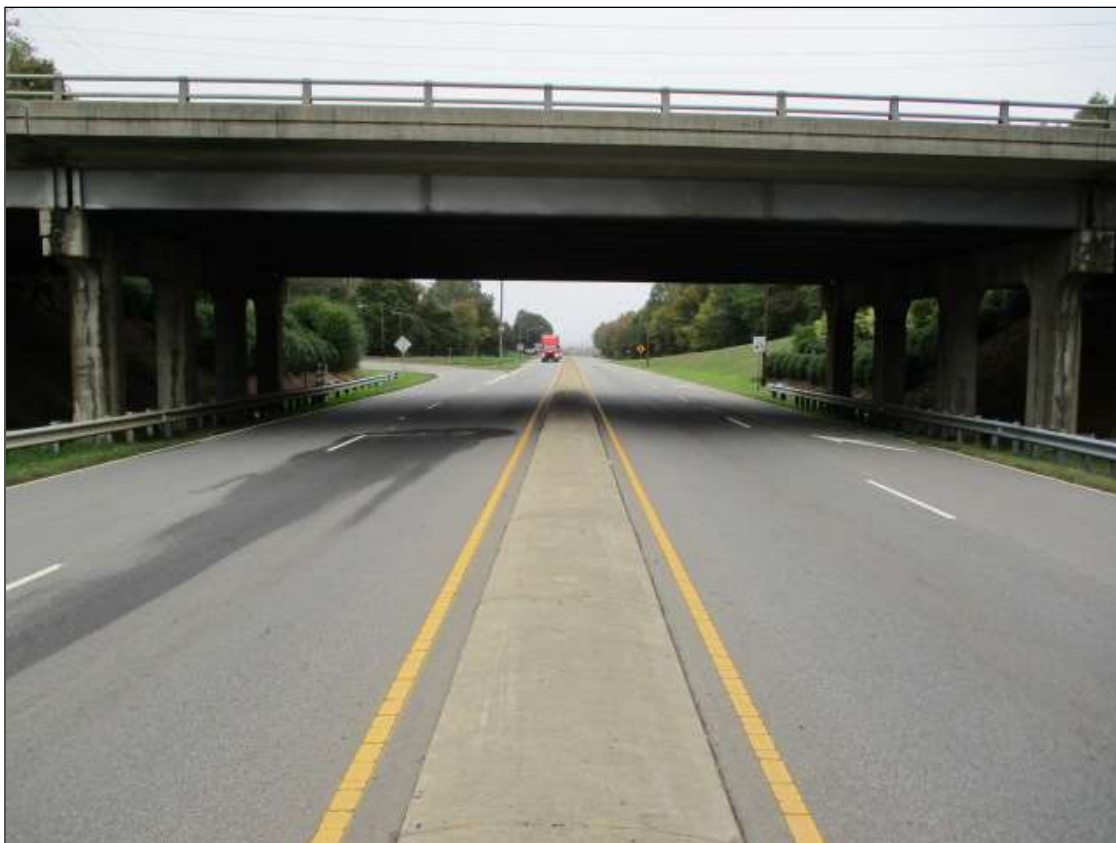
SOUTH ELEVATION OF SPAN 2
