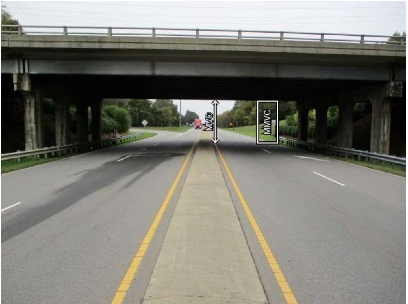
SPAN 2 NORTH BOUND LANE
