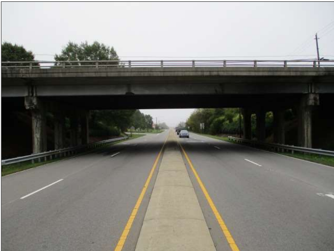
NORTH ELEVATION OF SPAN 2
