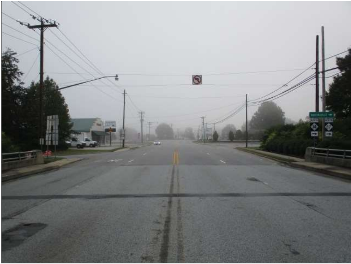
LOOKING EAST FROM BRIDGE
