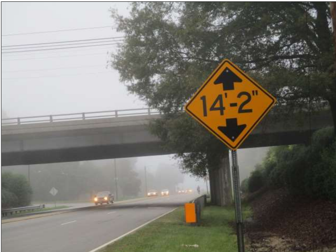
LOOKING CLEARANCE SIGN ON SOUTH SIDE AT 120' FROM BRIDGE
