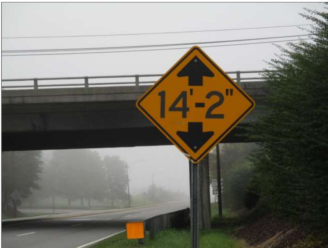
LOW CLEARANCE SIGN ON NORTH SIDE AT 100' FROM BRIDGE
