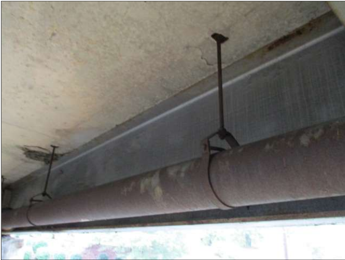
UTILITY IN BAY 8
