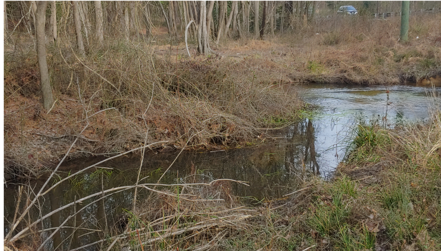
SOUTH APPROACH TO END BENT 1 LOOKING NORTH
