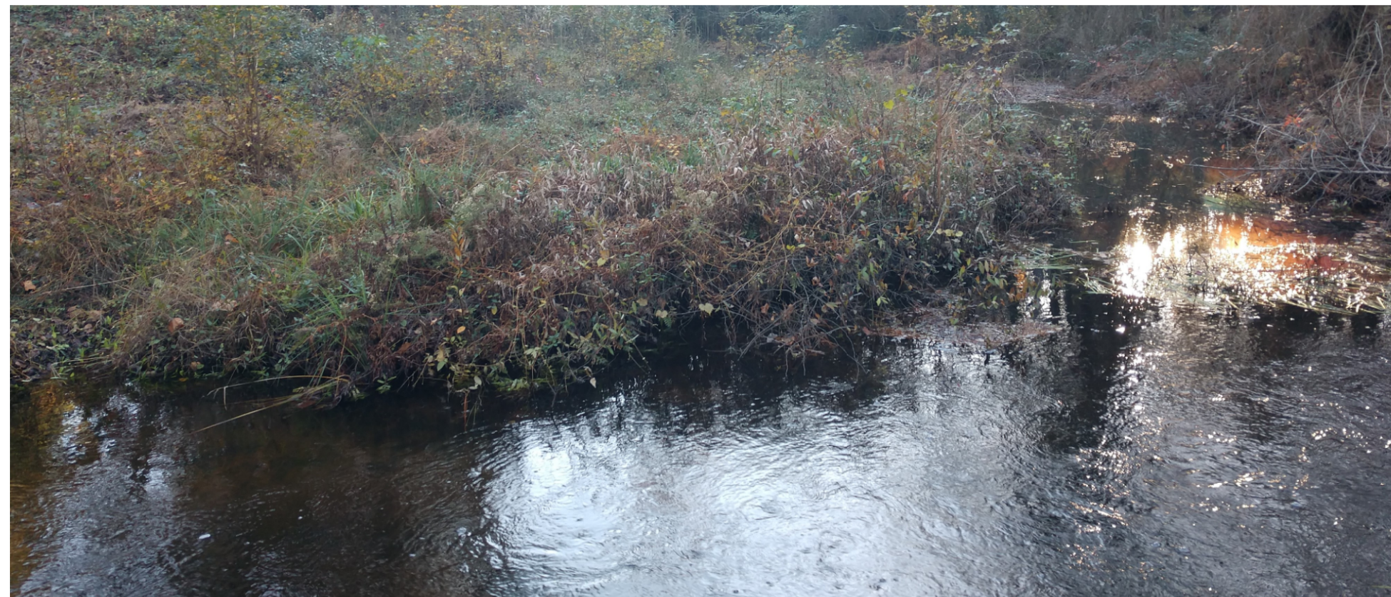
NORTH APPROACH TO END BENT 2 LOOKING SOUTH
