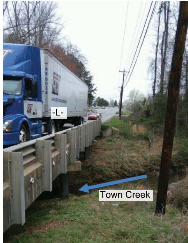
Photo 3: Looking South (Down-Station) along SR 2526 (Julian Road)
