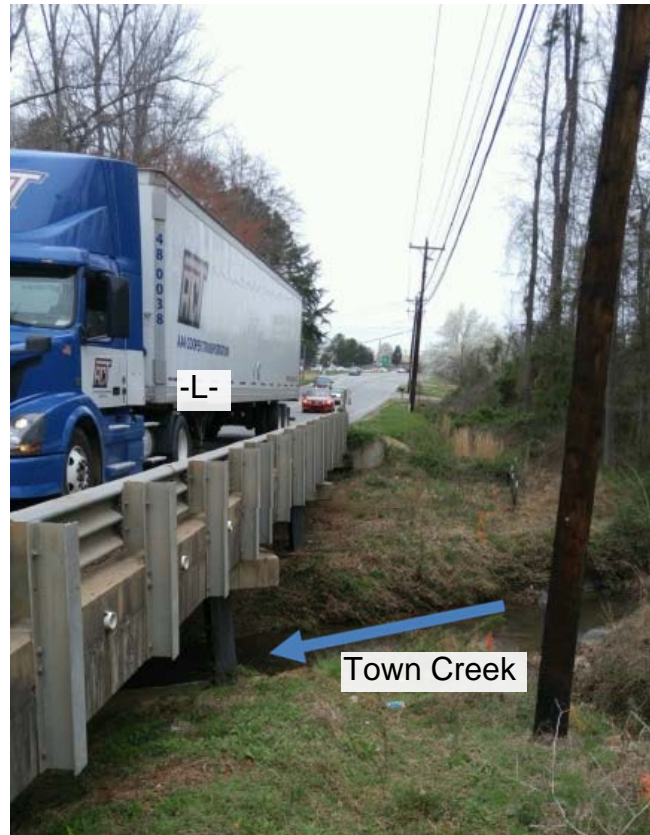
Photo 3: Looking South (Down-Station) along SR 2526 (Julian Road)
