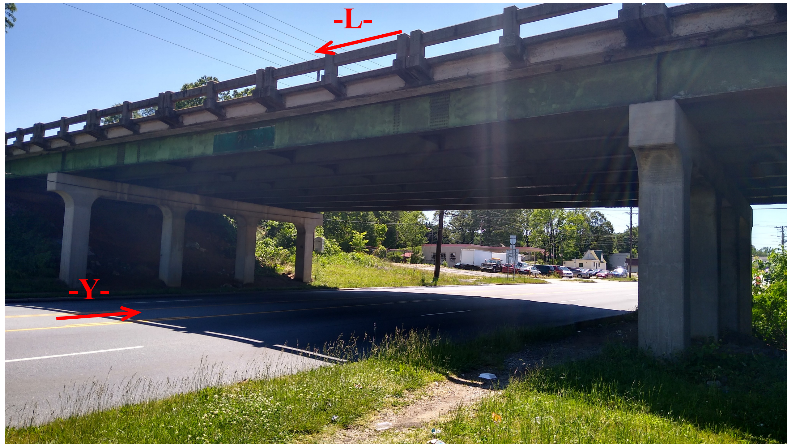
Looking East towards End Bent 2
