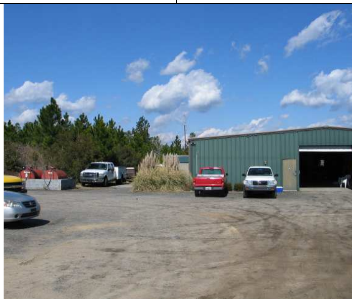
Site 35: Castle Bay Golf Course Maintenance Shop. View to the north.
