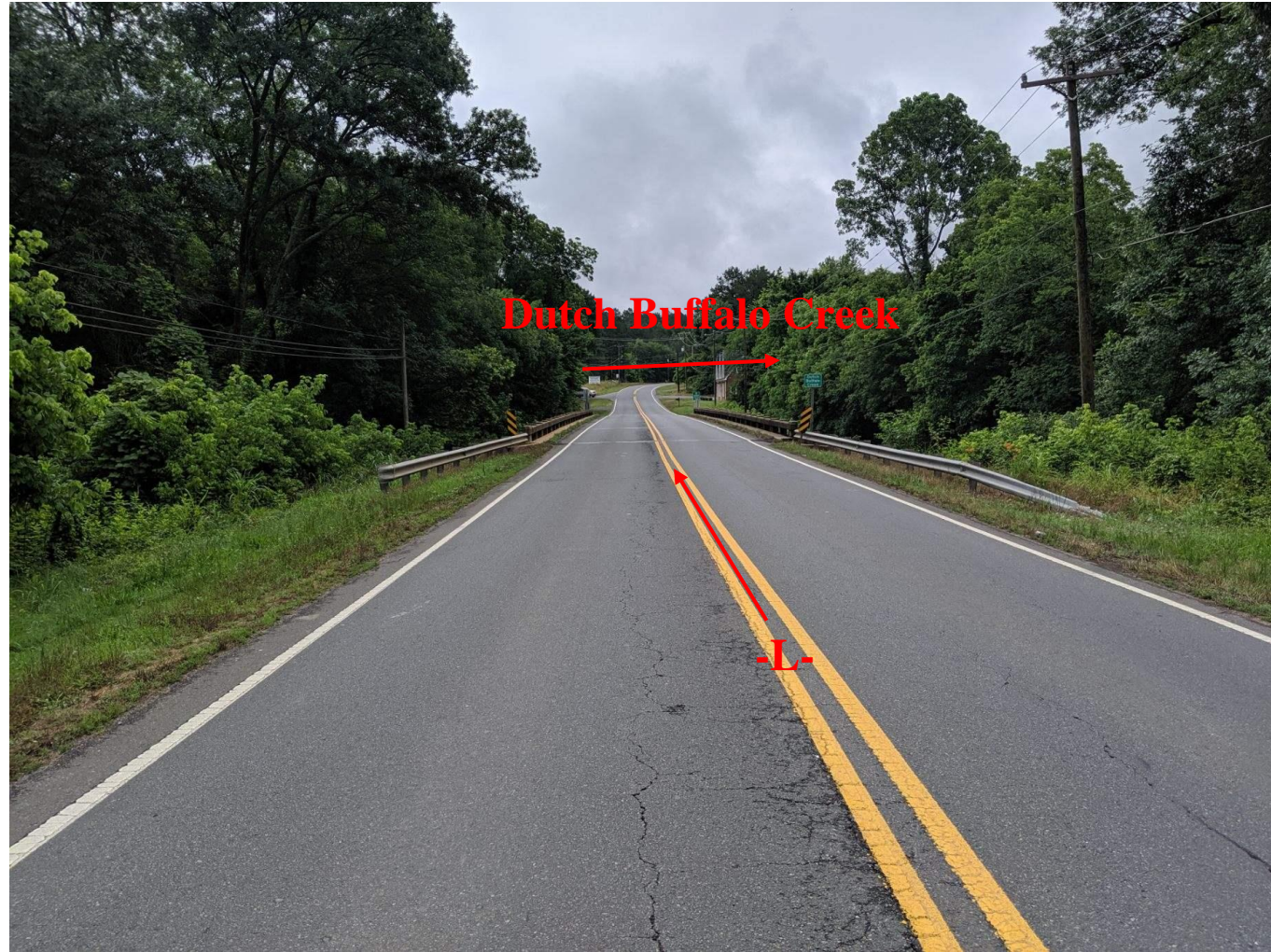
Photograph No. 1: Looking at End Bent 1 toward End Bent 2
