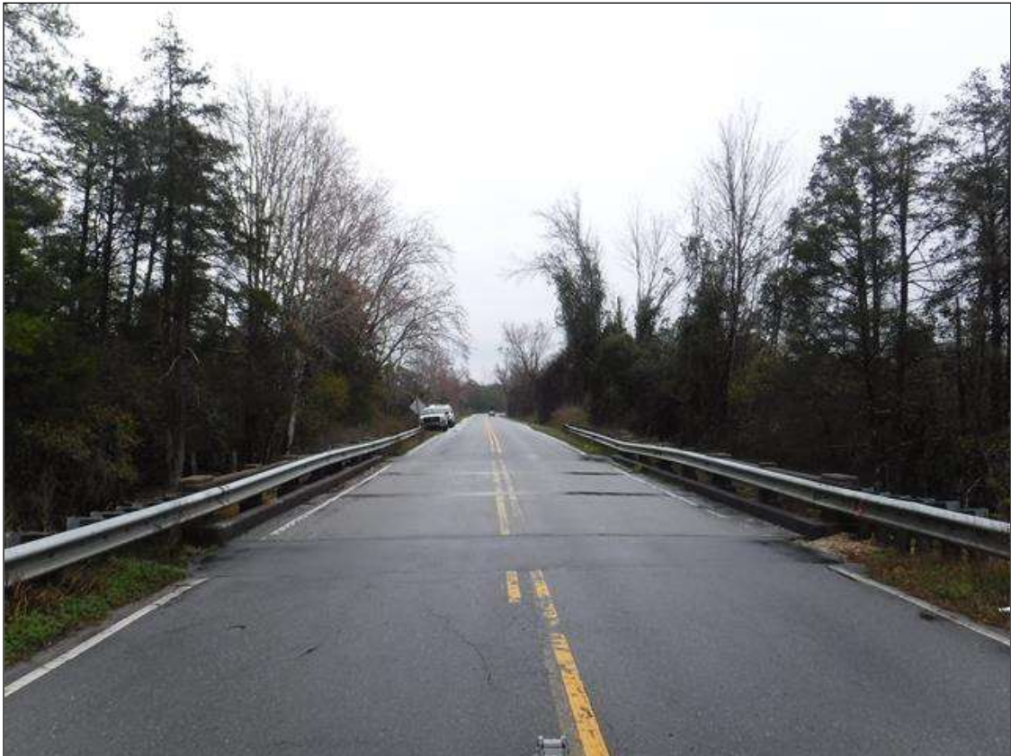
NORTH APPROACH, LOOKING SOUTH
