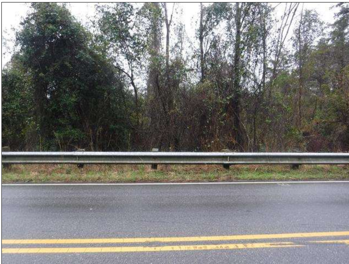
SOUTHWEST APPROACH GUARDRAIL POST SPACING AT MID LENGTH
