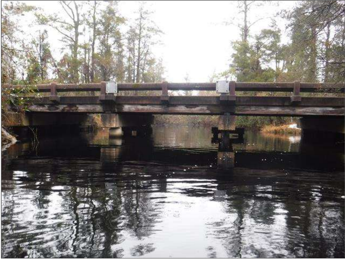
DOWNSTREAM PROFILE, LOOKING EAST
