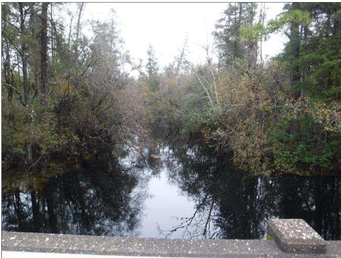
LOOKING UPSTREAM, EAST
