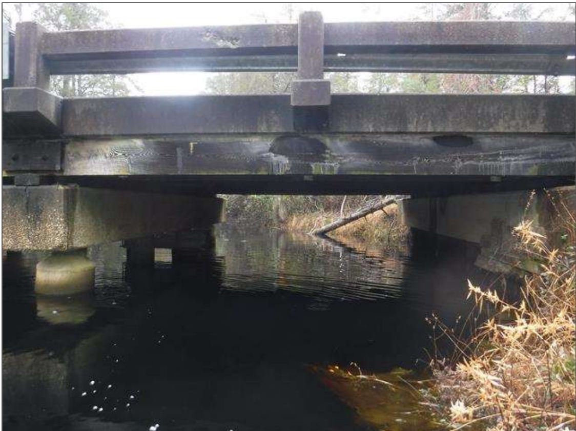
SPAN 3 UPSTREAM PROFILE, LOOKING WEST
