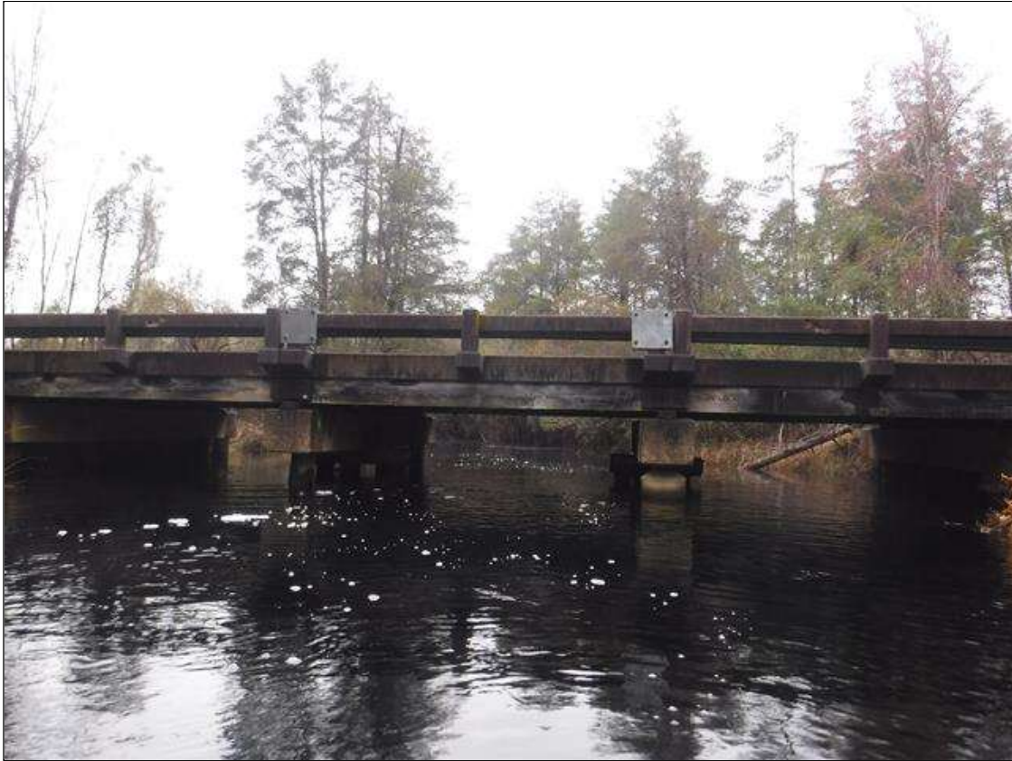
UPSTREAM PROFILE, LOOKING WEST
