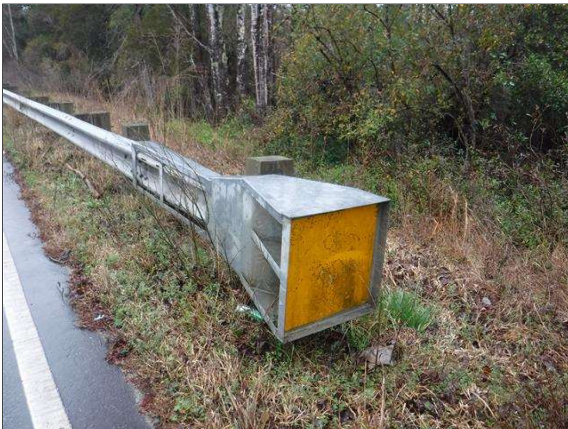
GUARDRAIL END TREATMENT AT SOUTHEAST CORNER, OTHERS SIMILAR
