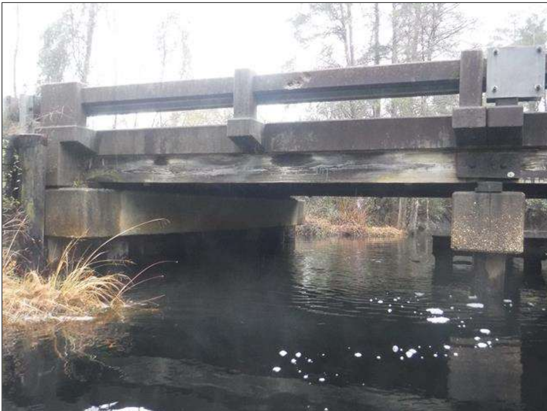
SPAN 1 UPSTREAM PROFILE, LOOKING WEST
