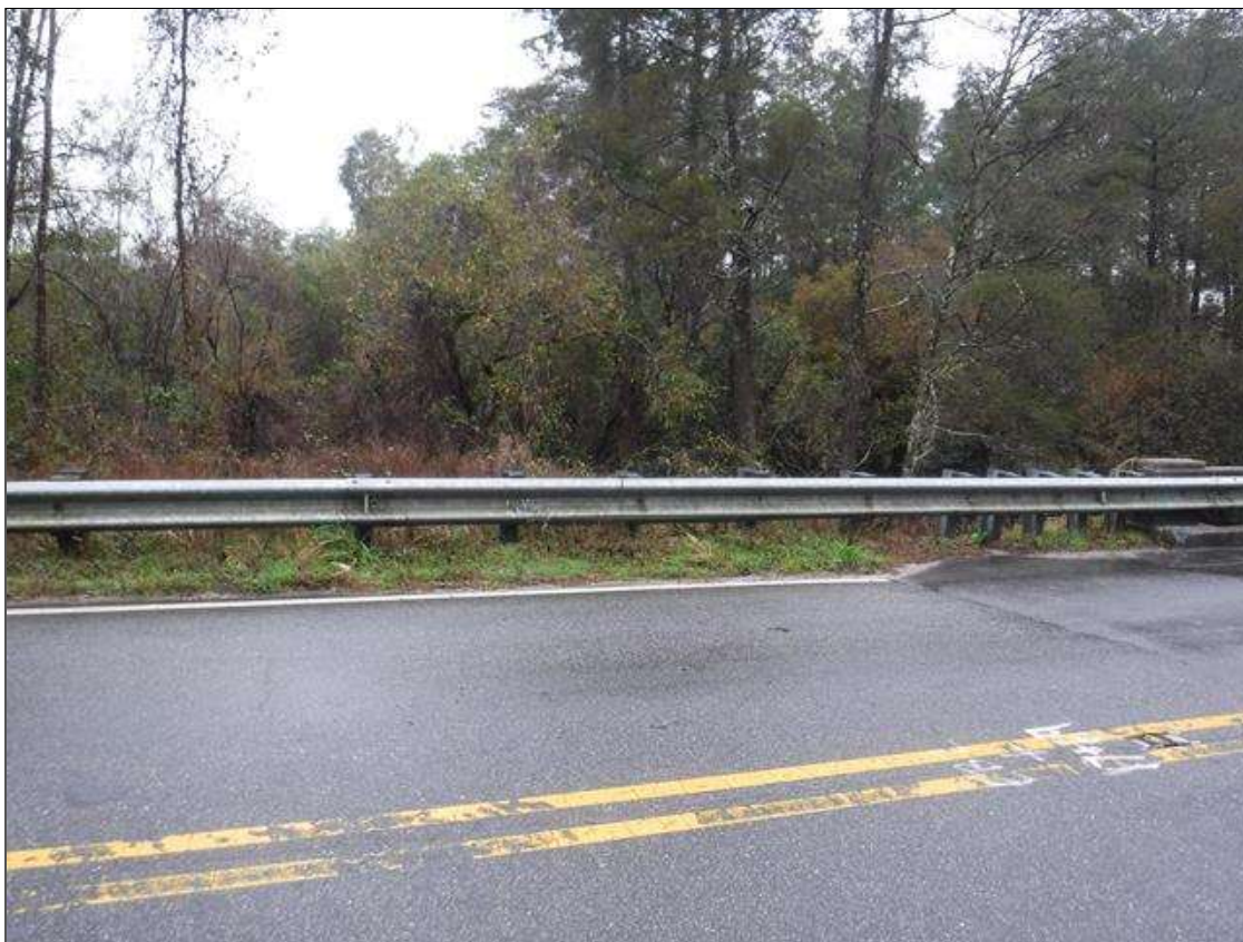
SOUTHWEST APPROACH GUARDRAIL POST SPACING AT BRIDGE
