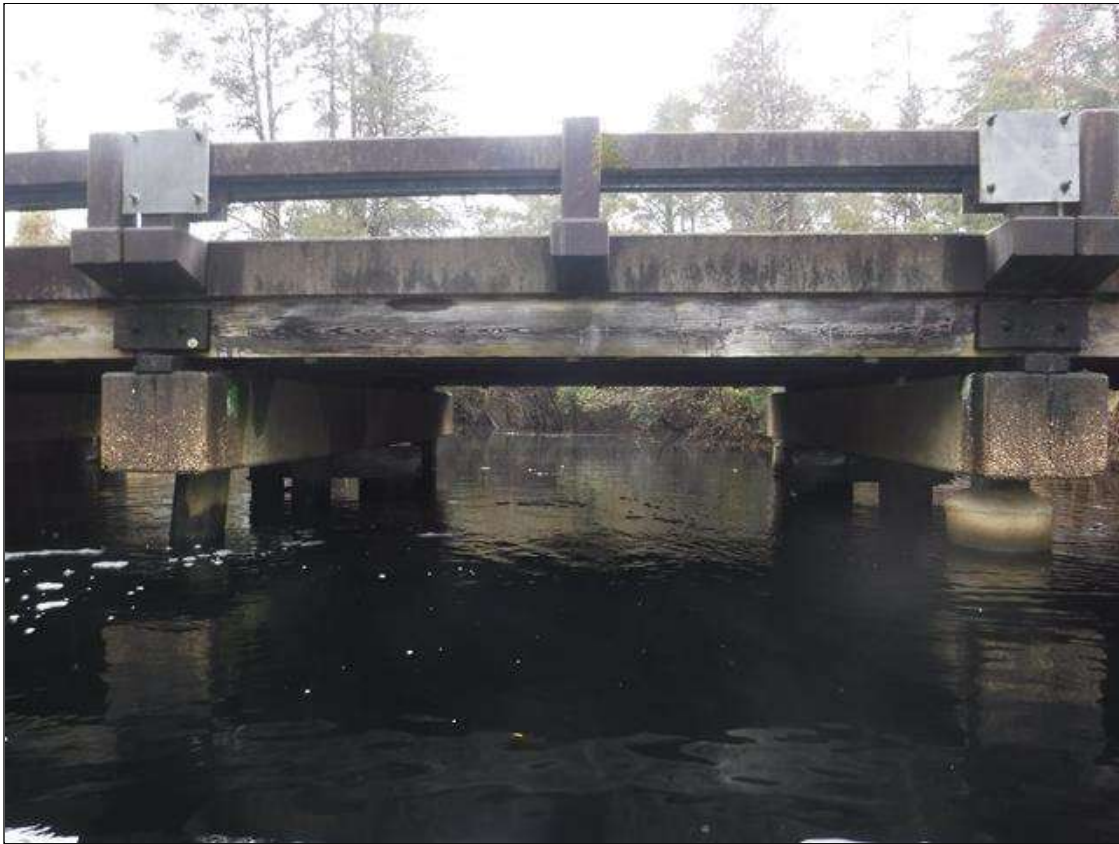
SPAN 2 UPSTREAM PROFILE, LOOKING WEST
