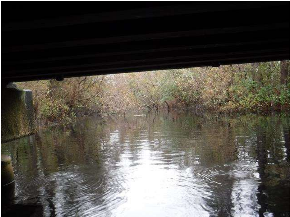
LOOKING UPSTREAM, EAST
