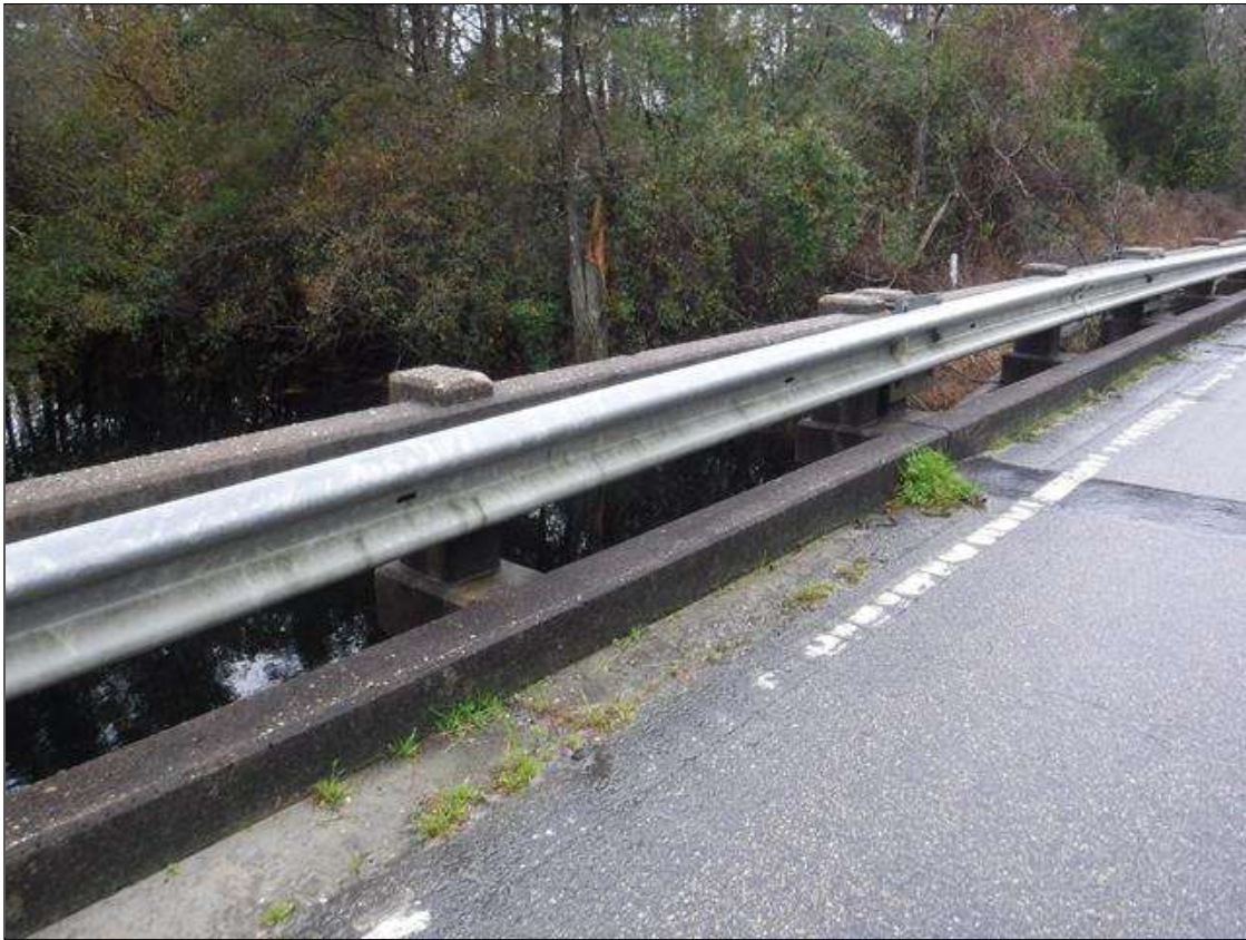
LEFT RAIL, RIGHT RAIL SIMILAR
