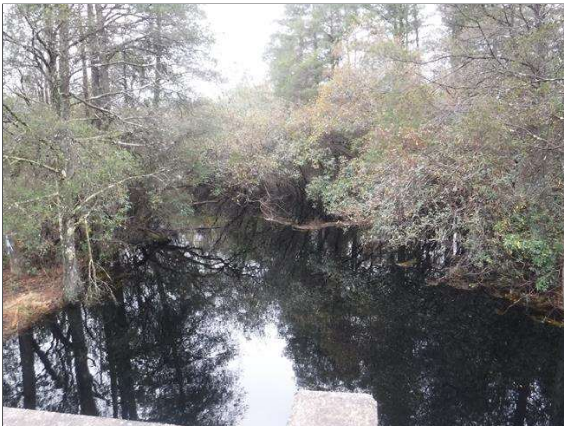
LOOKING DOWNSTREAM, WEST
