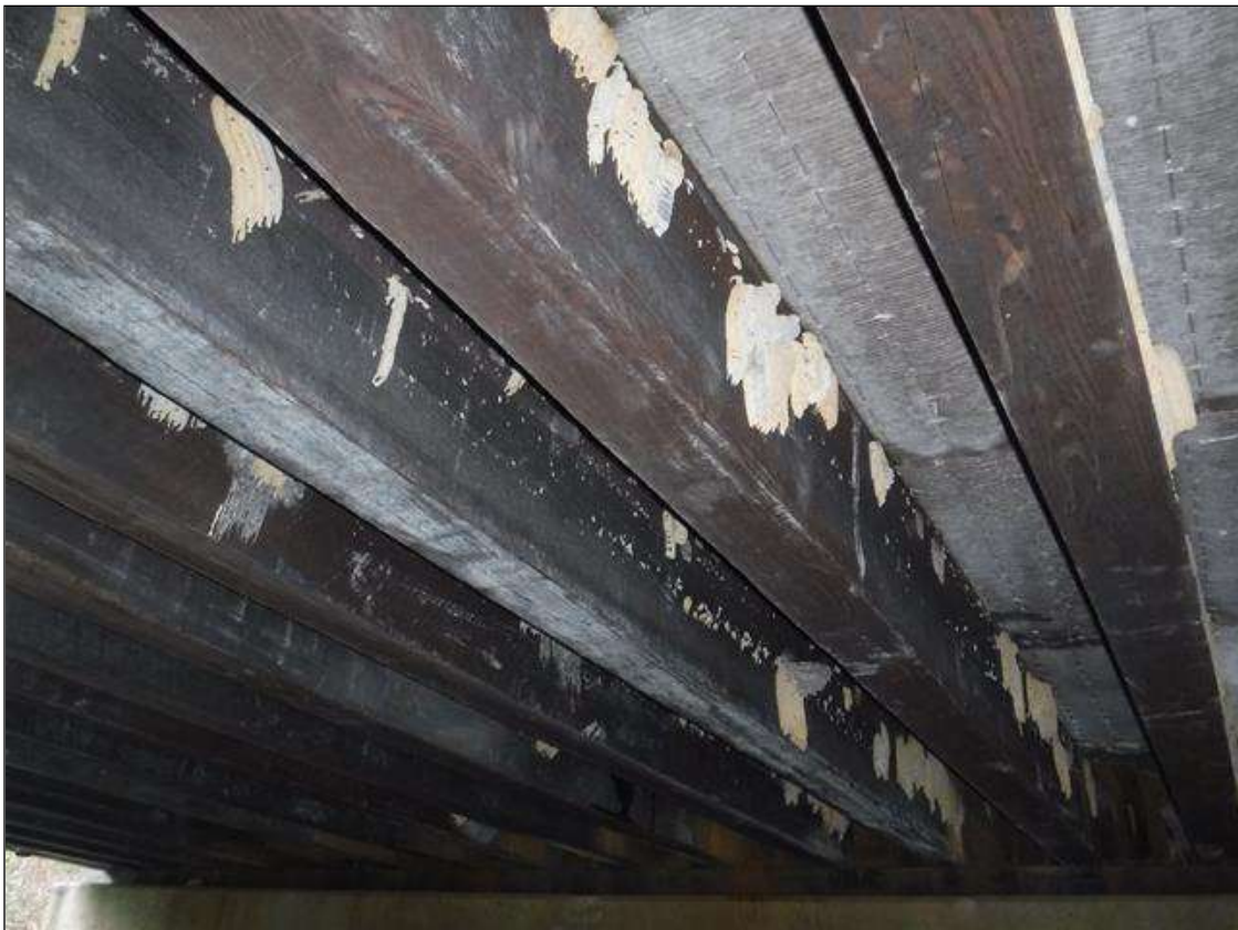
SPAN 2 UNDERDECK, OTHERS SIMILAR
