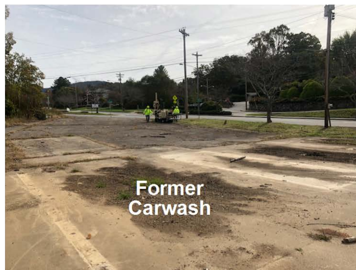
Drillers setting up on boring B-17. Footprint of former carwash is in the foreground.
