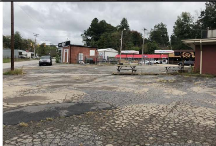
3. View along north side of property from the northwest corner.
