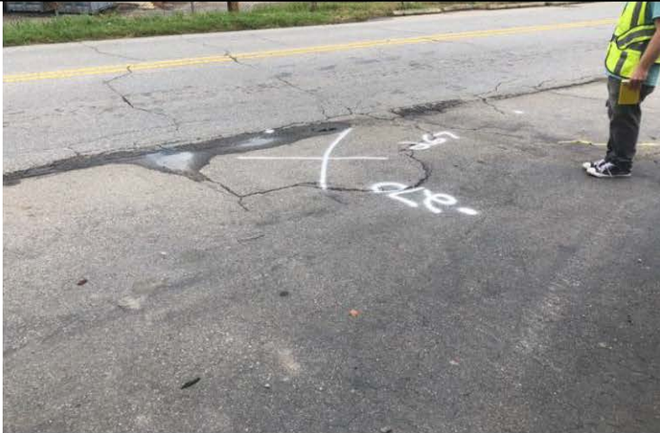
2. Magnetic anomaly A near reported location of former heating oil UST off west corner of building. Natural gas line runs into building to the north of this anomaly .
