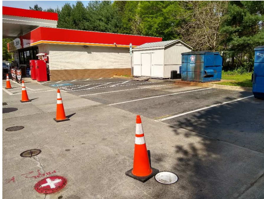
A. Photograph of edge of known USTs and part of study area on east side of the gas station, looking west.
