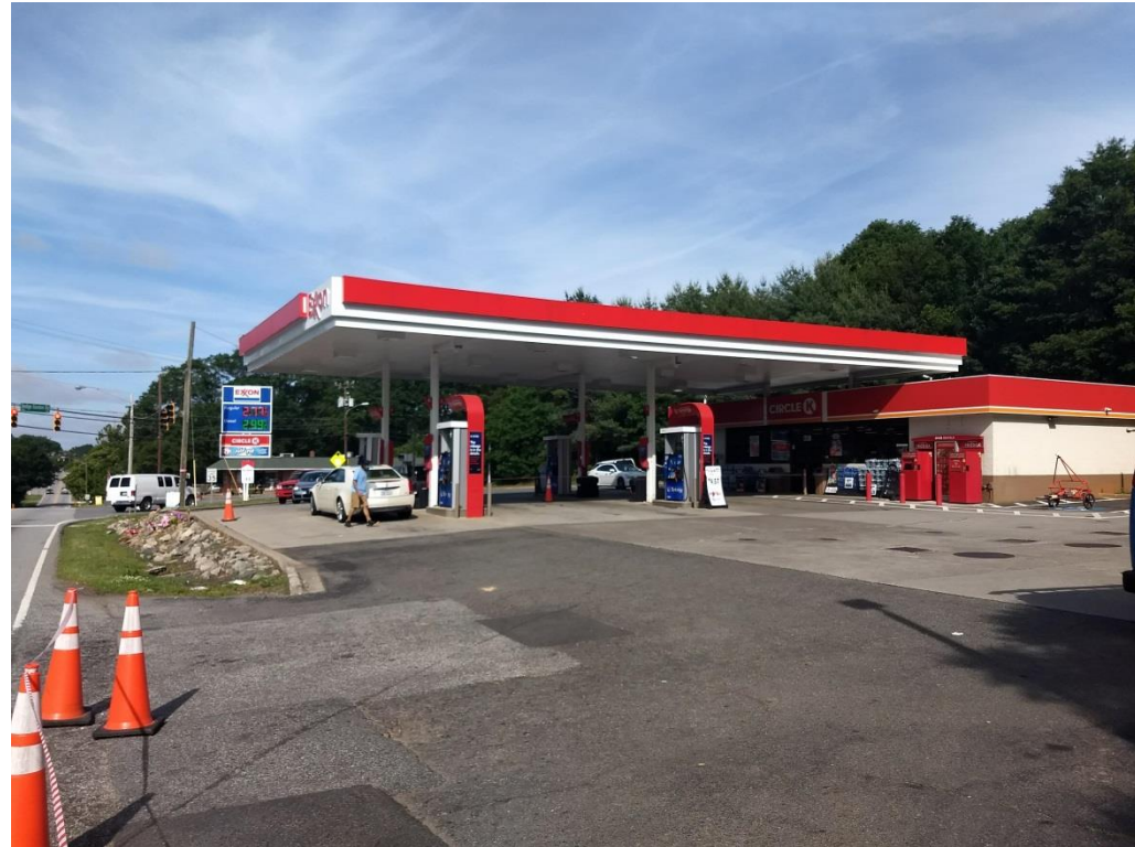
a. Photo from northeast side of site looking southwest.
