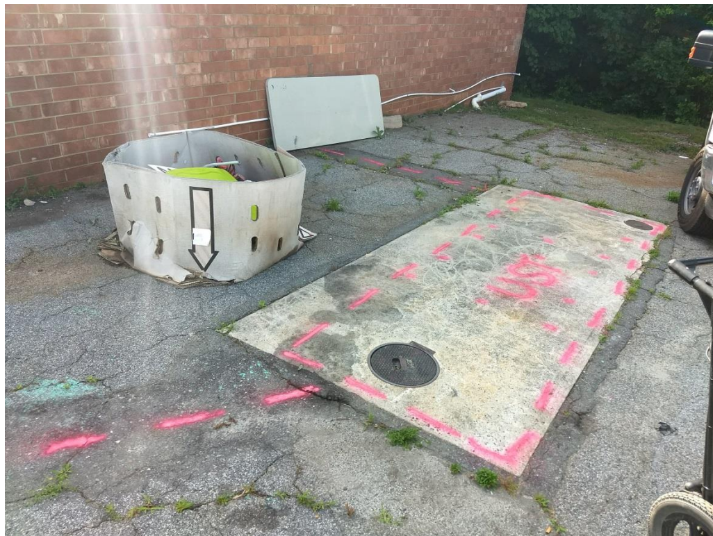
c. Photo of marked probable UST.
