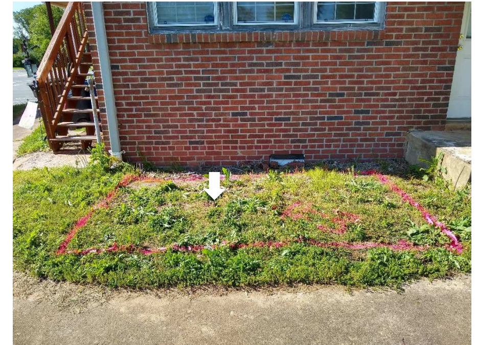
F. Photograph of rear of residence showing marked location of probable abandoned heating oil UST with apparent vent or fill pipe indicated by white arrow.
