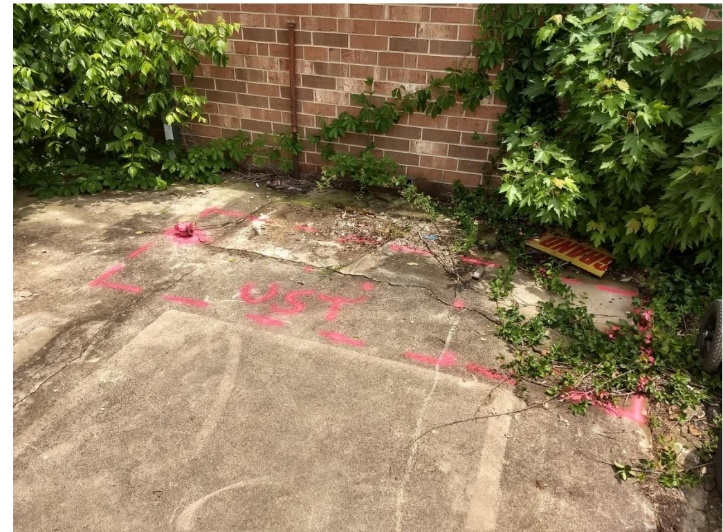
d. Photo of marked probable UST.
