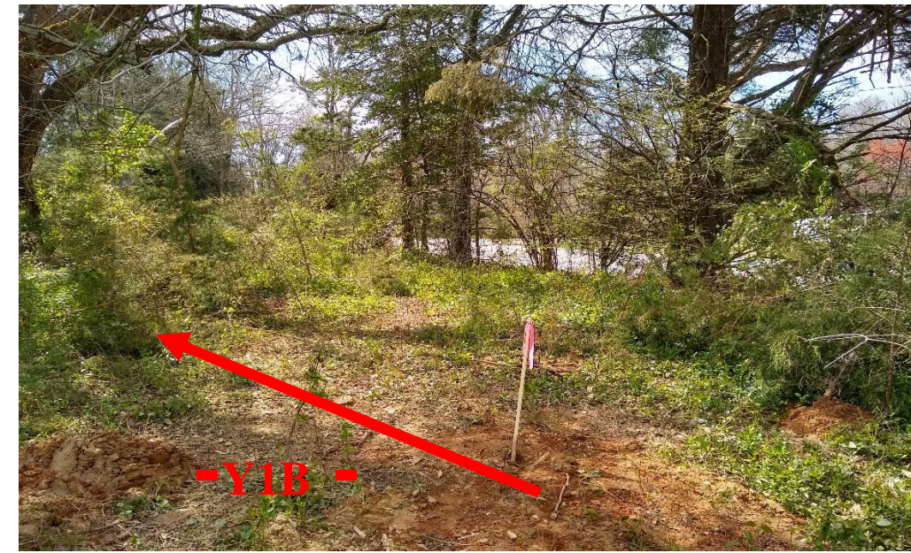
View Along Bent 1 Looking Left to Right
