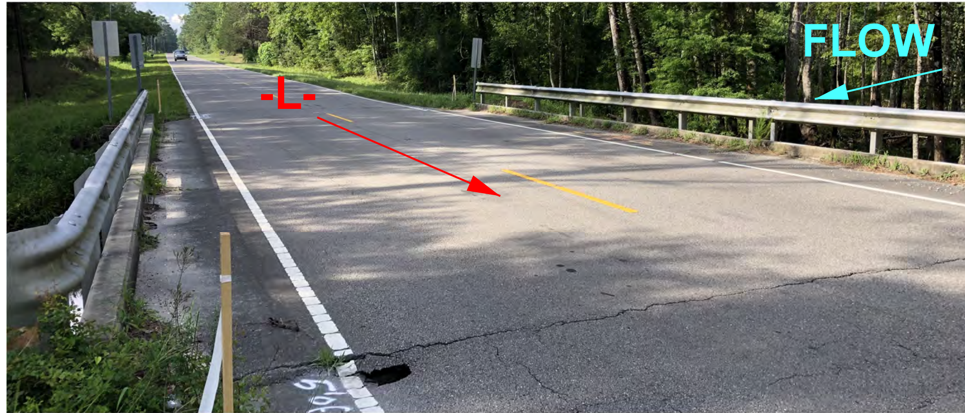
LOOKING SOUTH FROM END BENT 2 TOWARD END BENT 1
