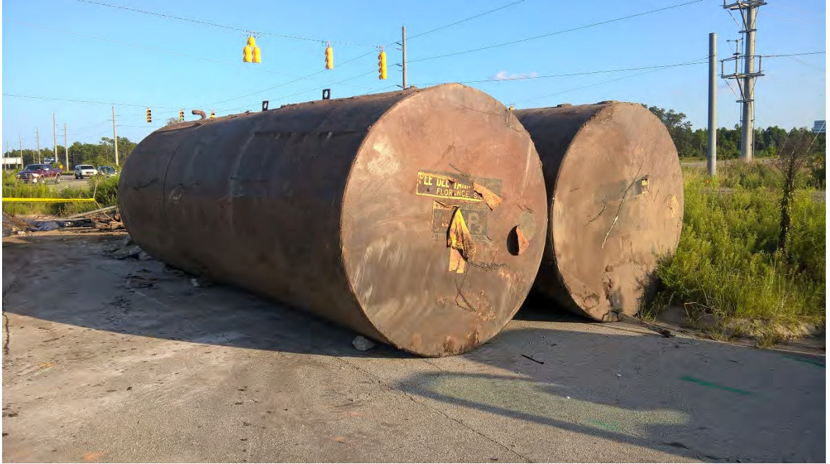
9/19: View of UST-2 (right) and UST-1 (left).
