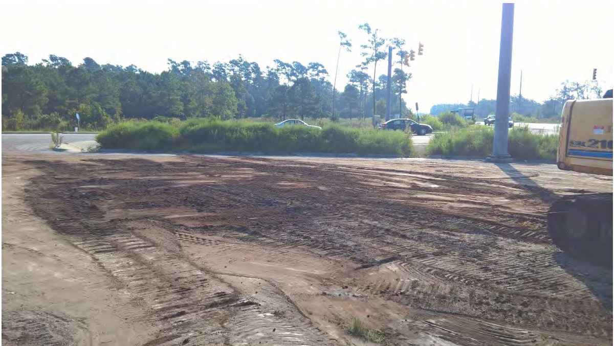
9/21: View of backfilled excavation.
