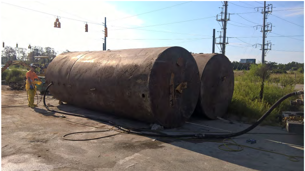
9/20: View of cleaning of UST-1 to remove vapors for transport.
