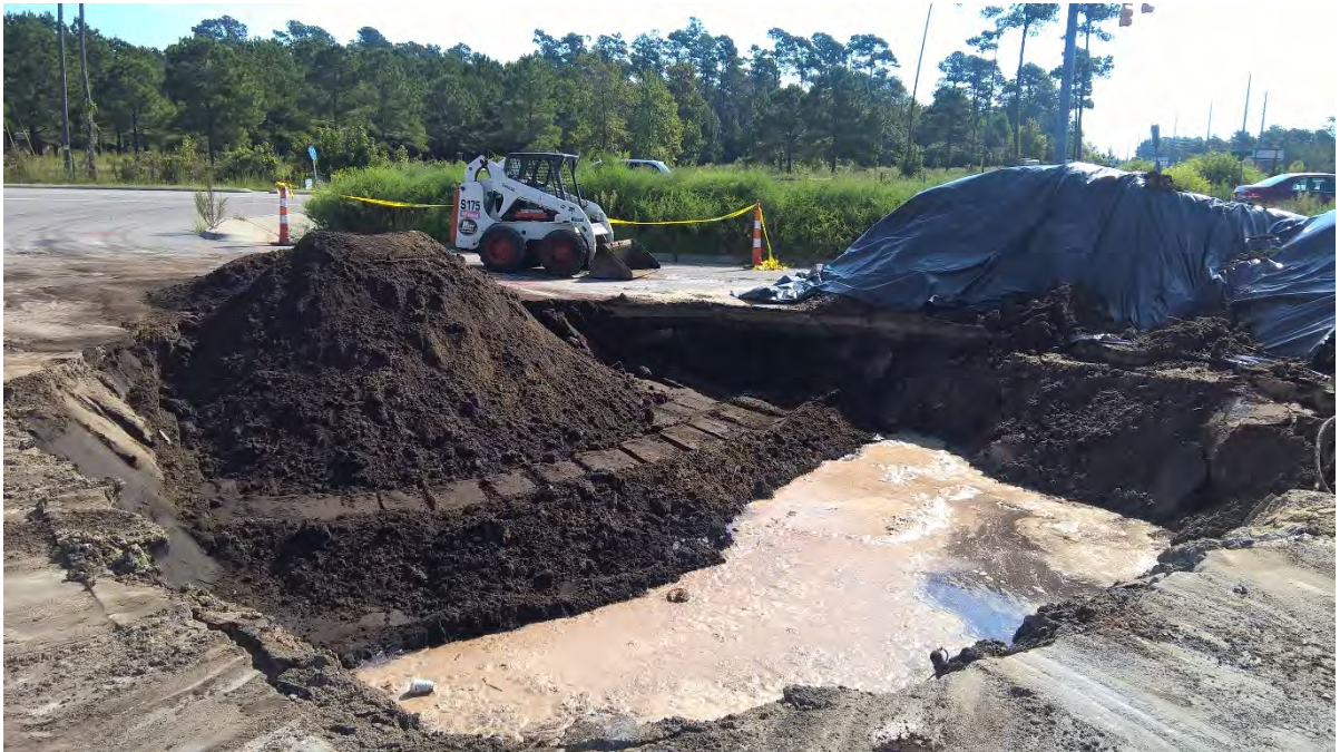
9/20: View of backfilling.
