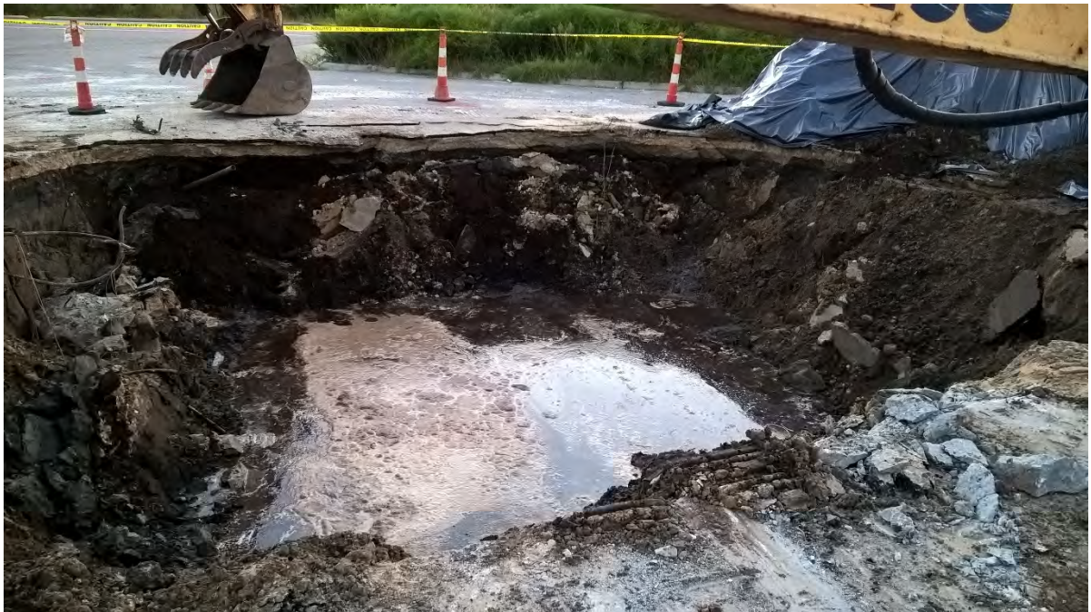
9/19: View of groundwater in the UST basin.
