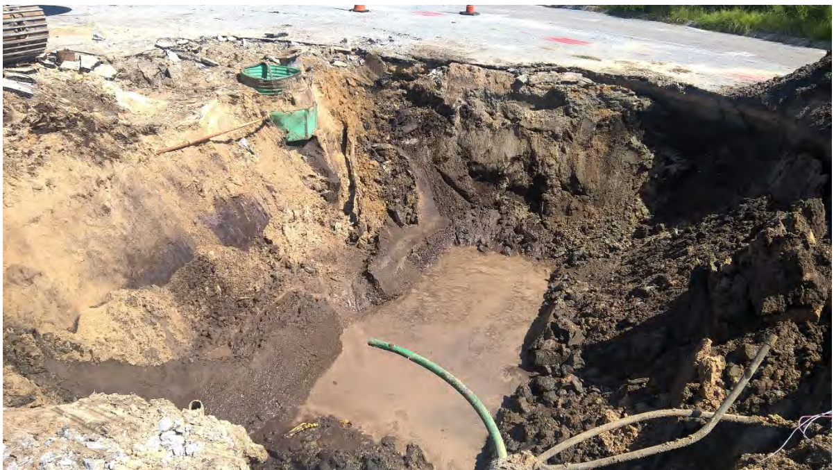
9/19: Groundwater observed in the excavation.
