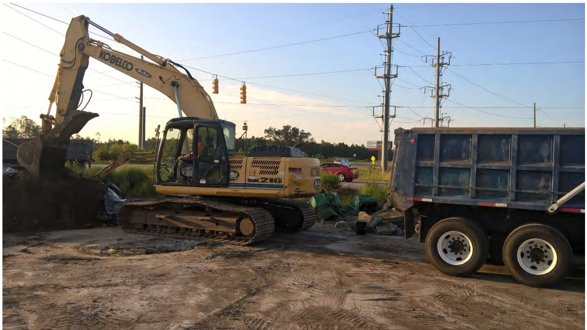
9/20: View of removing excavated soil.
