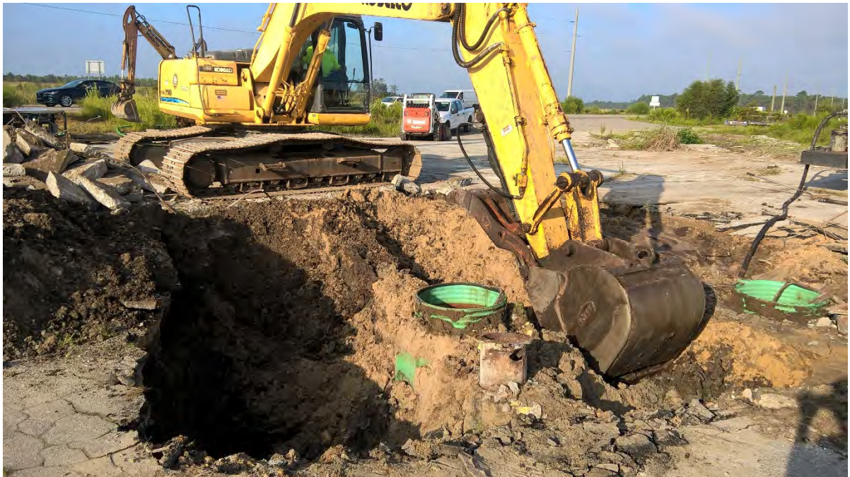
9/19: Excavating around USTs.
