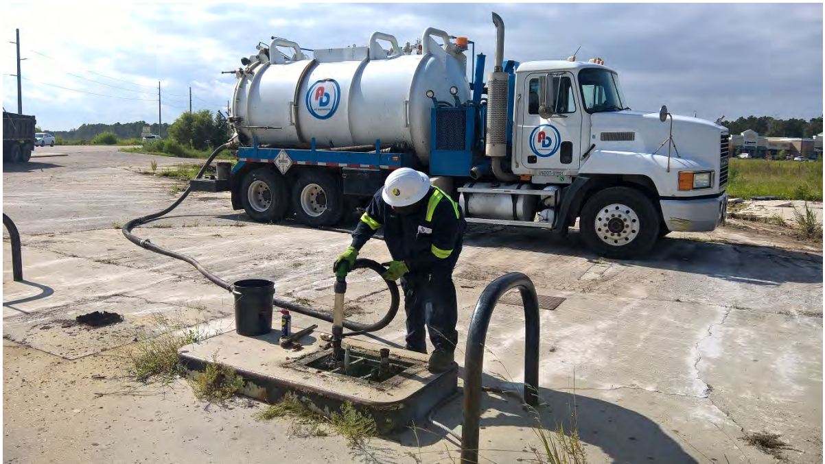
9/18: Removing residual liquid from the product lines.
