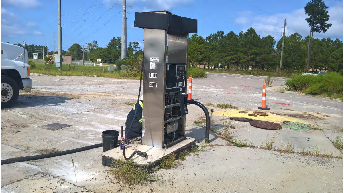
9/18: Removing dispenser pumps.
