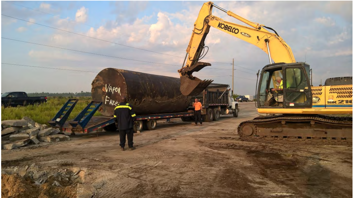
9/21: Removal of UST-2 from the site.
