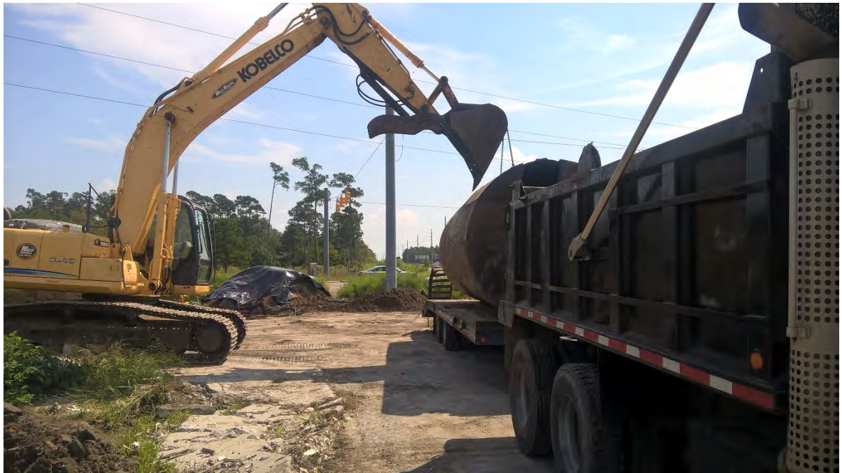
9/20: View of removal of UST-1 from the site.
