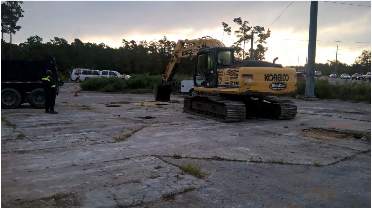
9/19: Removing concrete over USTs.
