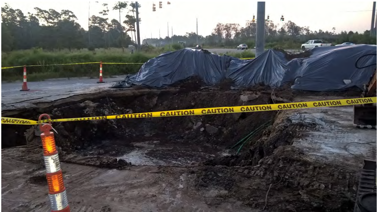
9/19: View of soil temporarily stockpiled onsite.
