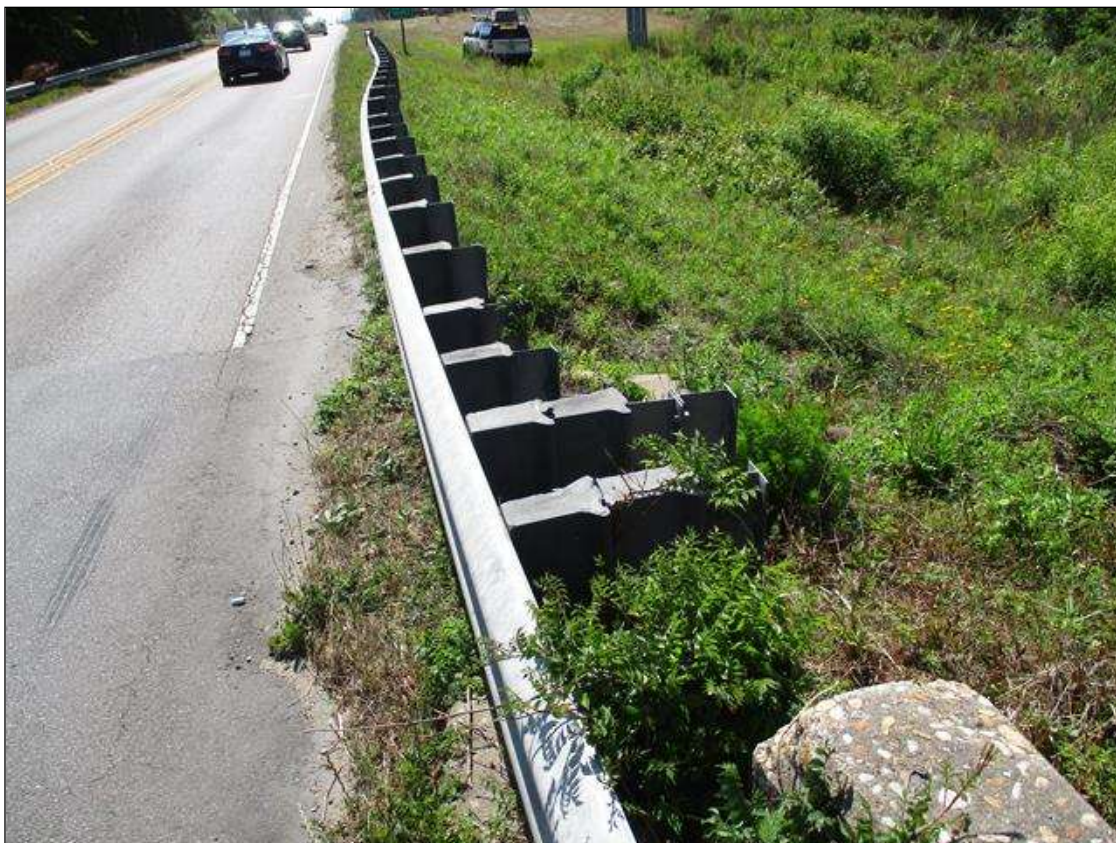
SIMILAR GUARDRAIL POST SPACES ( SOUTHWEST SHOWN )
