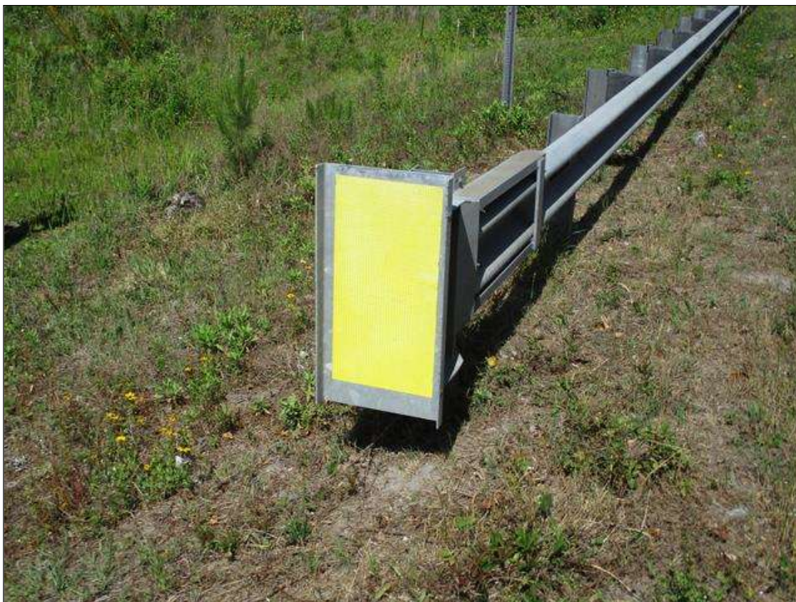
SOUTHWEST GUARDRAIL END TERMINAL ( SOUTHEAST , NORTHWEST SIMILAR )
