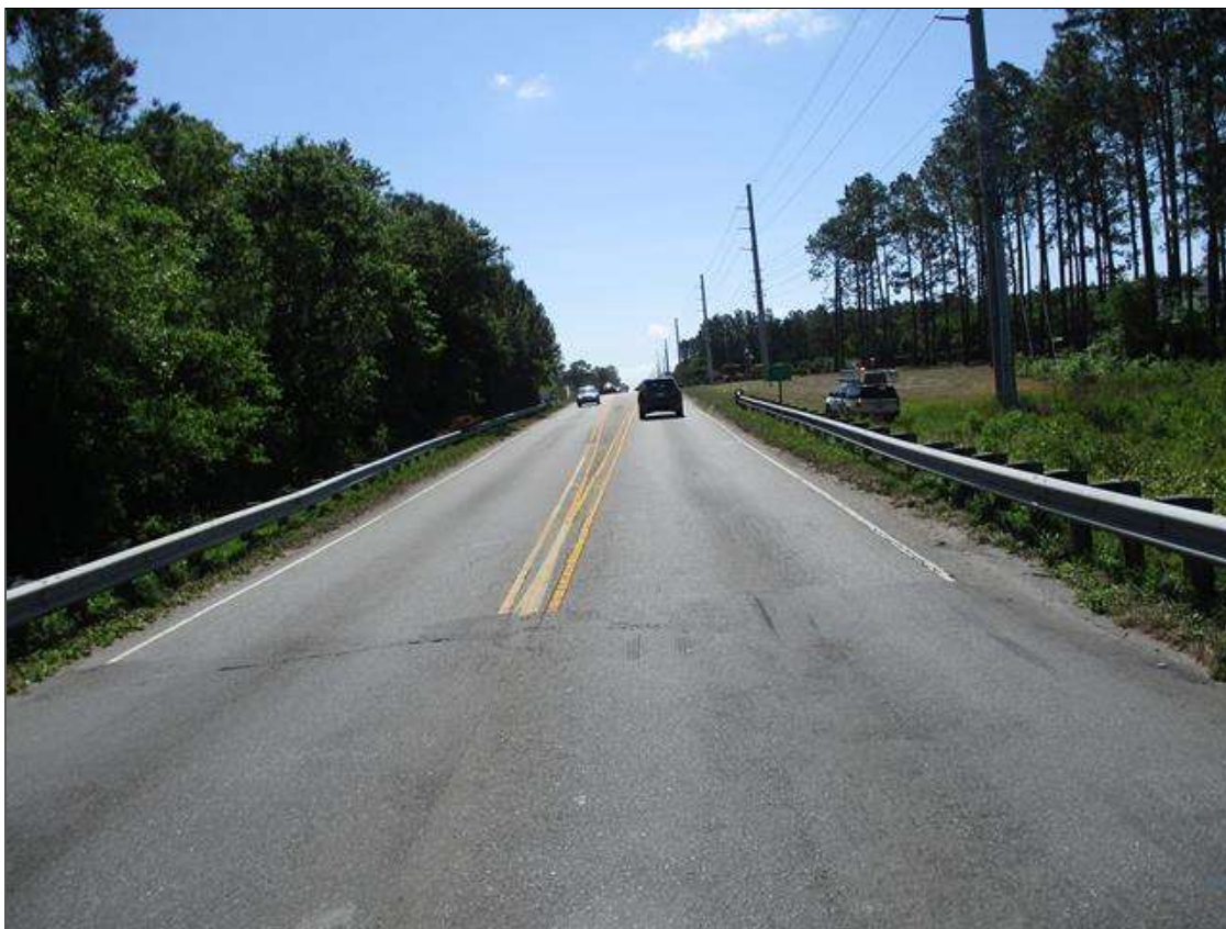
LOOKING SOUTH OFF STRUCTURE
