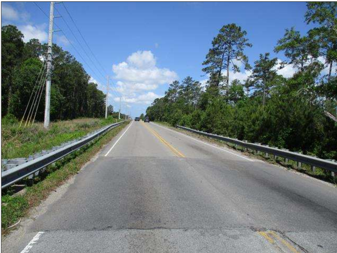
LOOKING NORTH OFF STRUCTURE
