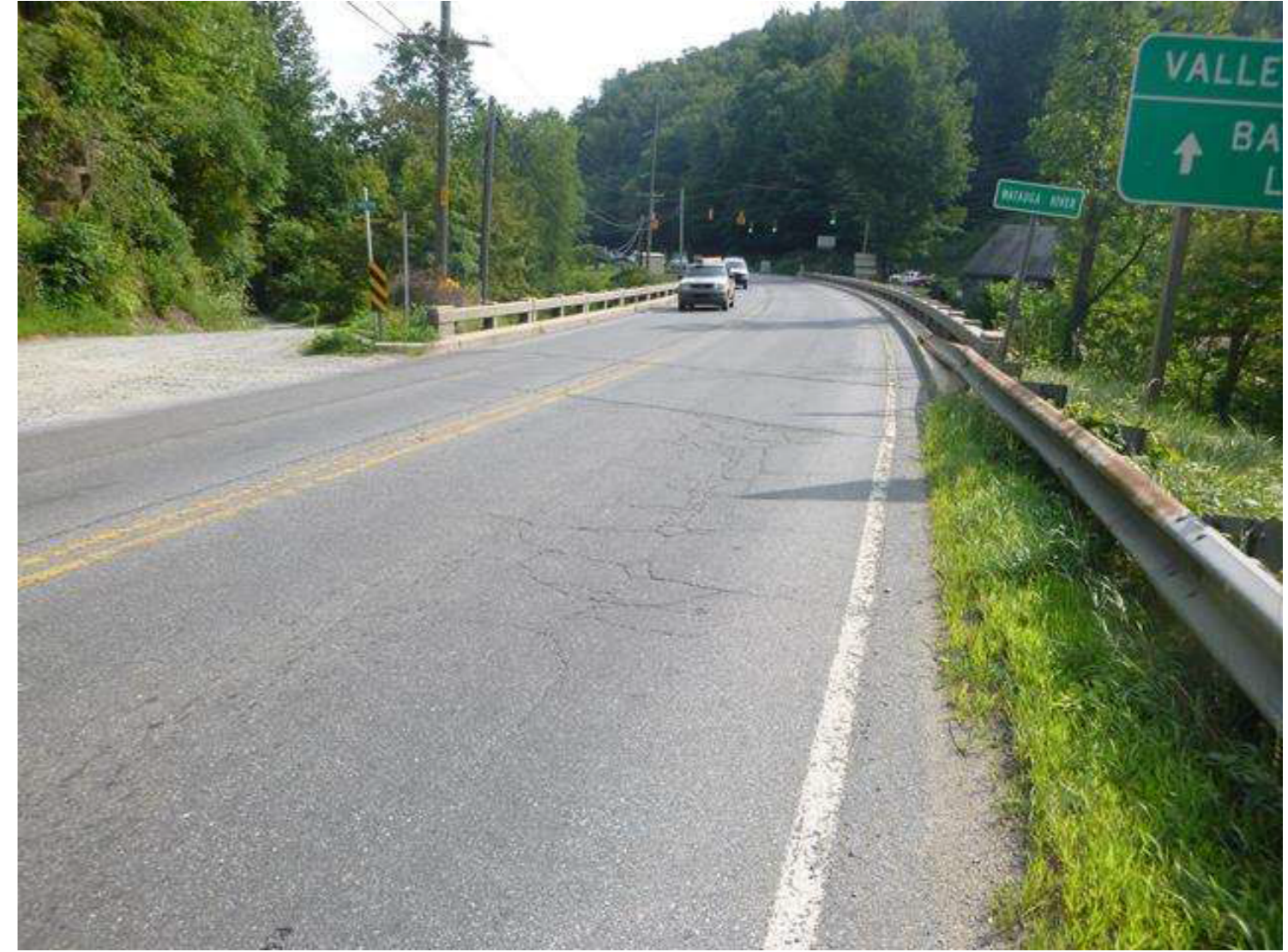
View along existing NC 105, facing South
