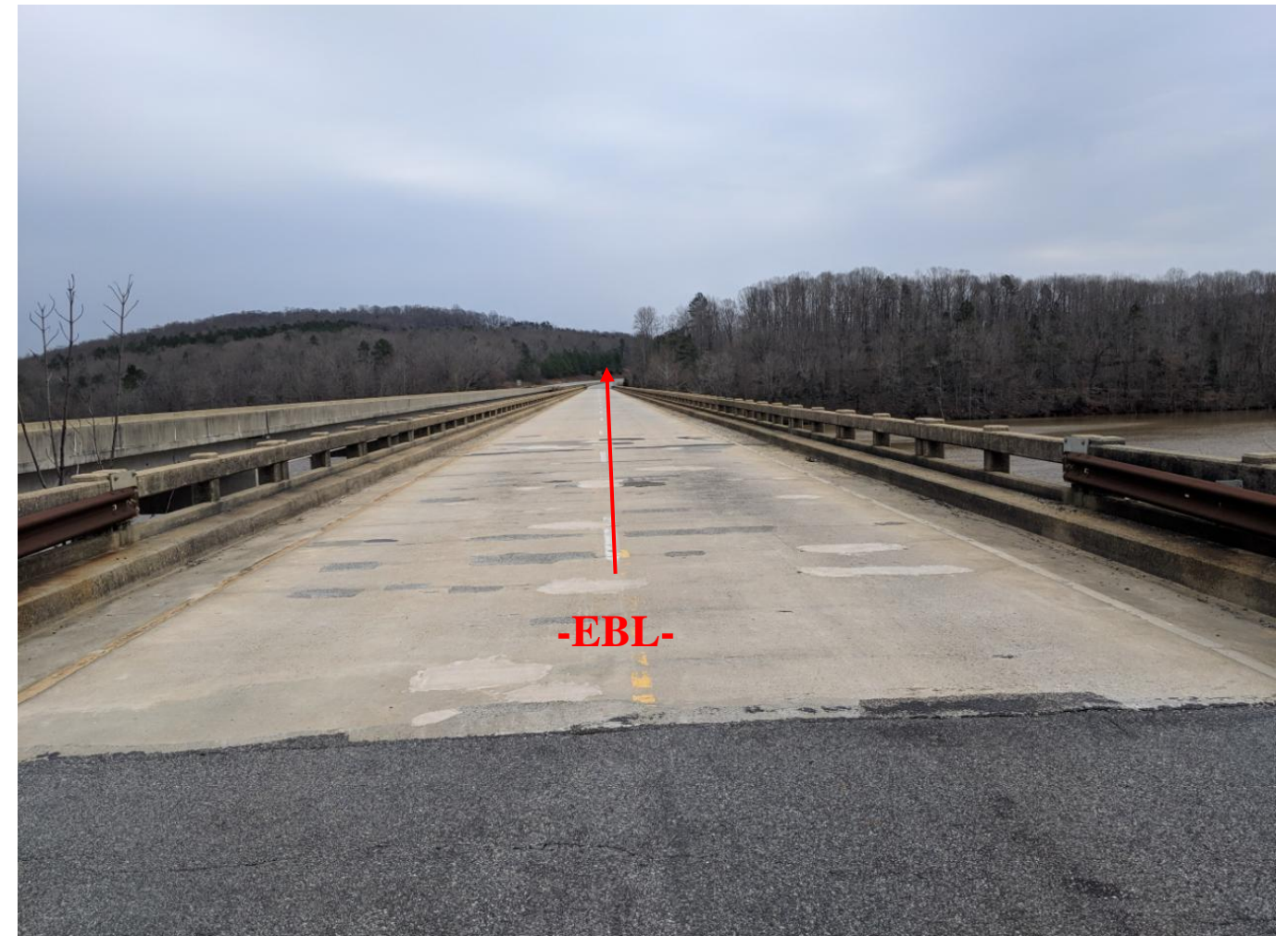
Photograph No. 2: Looking at End Bent 1 to End Bent 2
