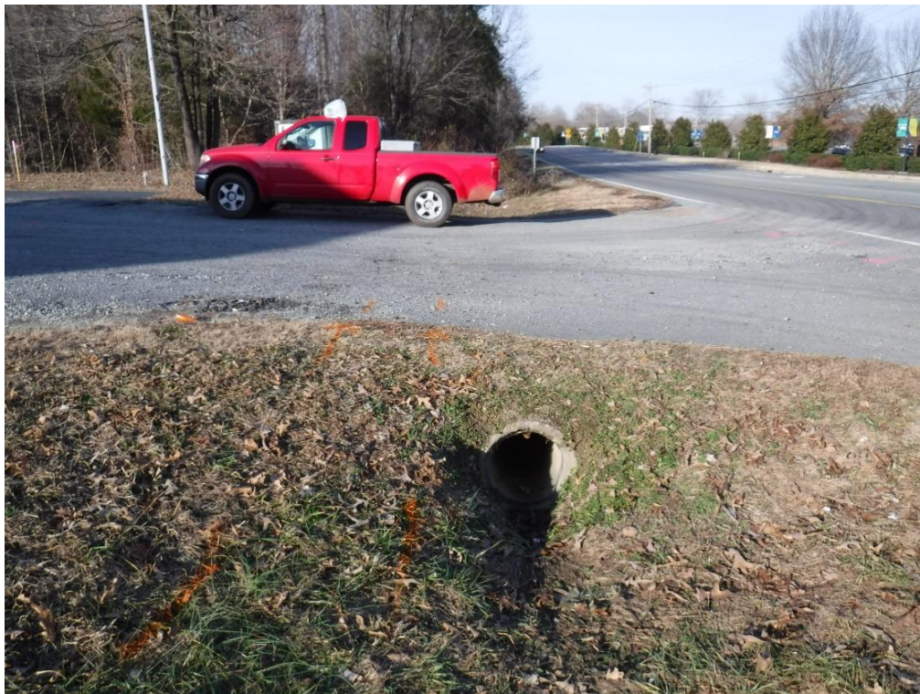
Photo 8: Looking North – Reinforced concrete storm drain culvert and stationary vehicle
