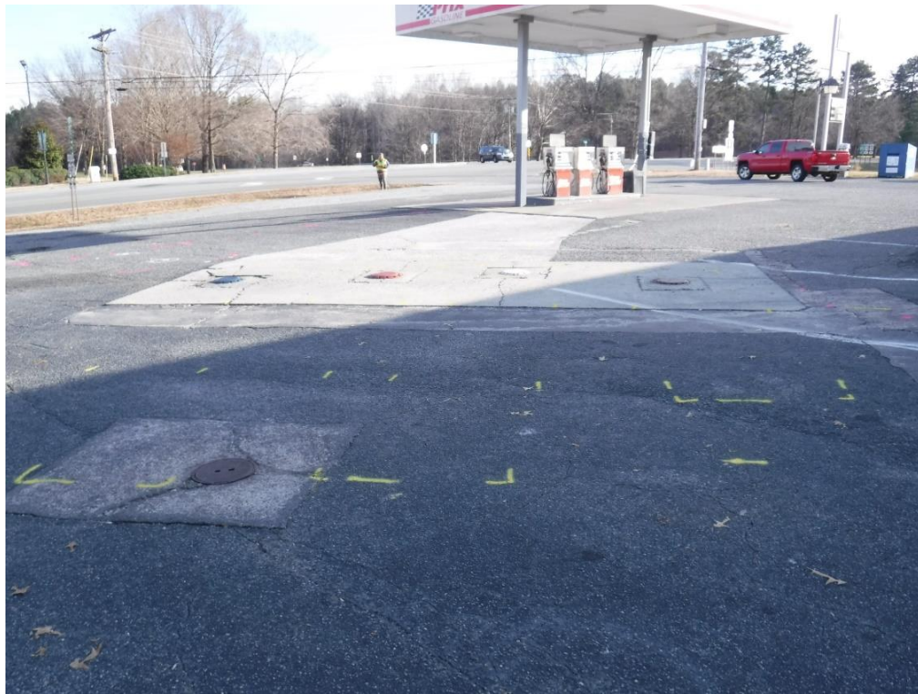
Photo 1: Looking South – Four Known UST's with approximate extents in yellow
