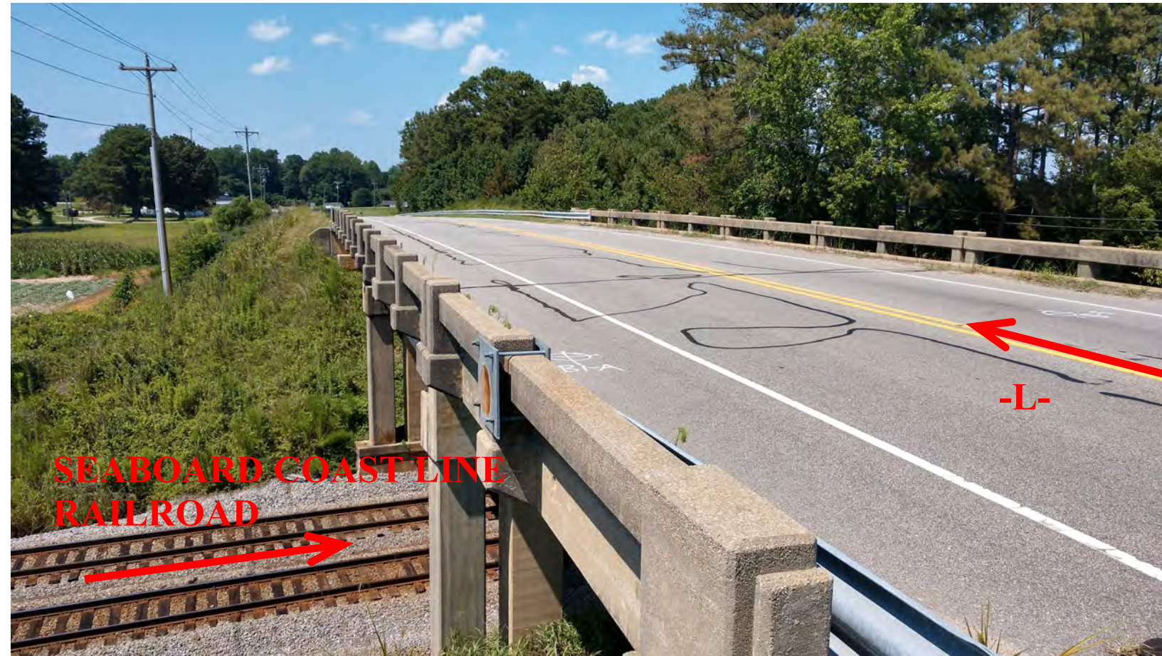
Looking North along -L- from End Bent No. 1
