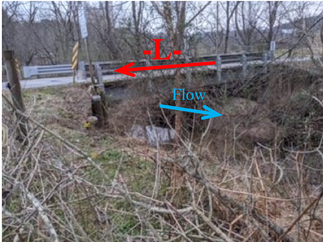
Looking South From End Bent 2
