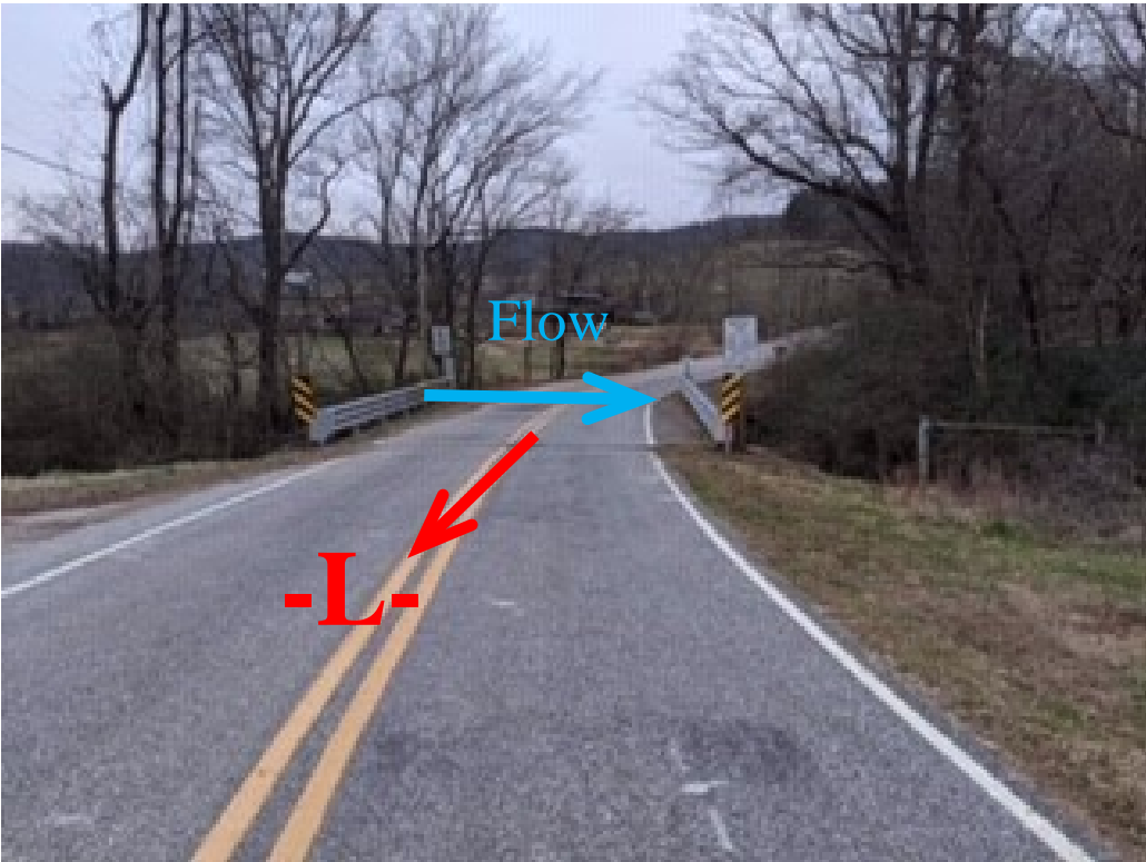
Looking South Toward End Bent 1
