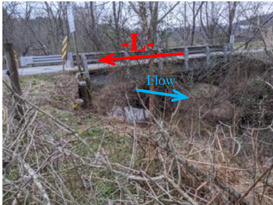
Looking South From End Bent 2
