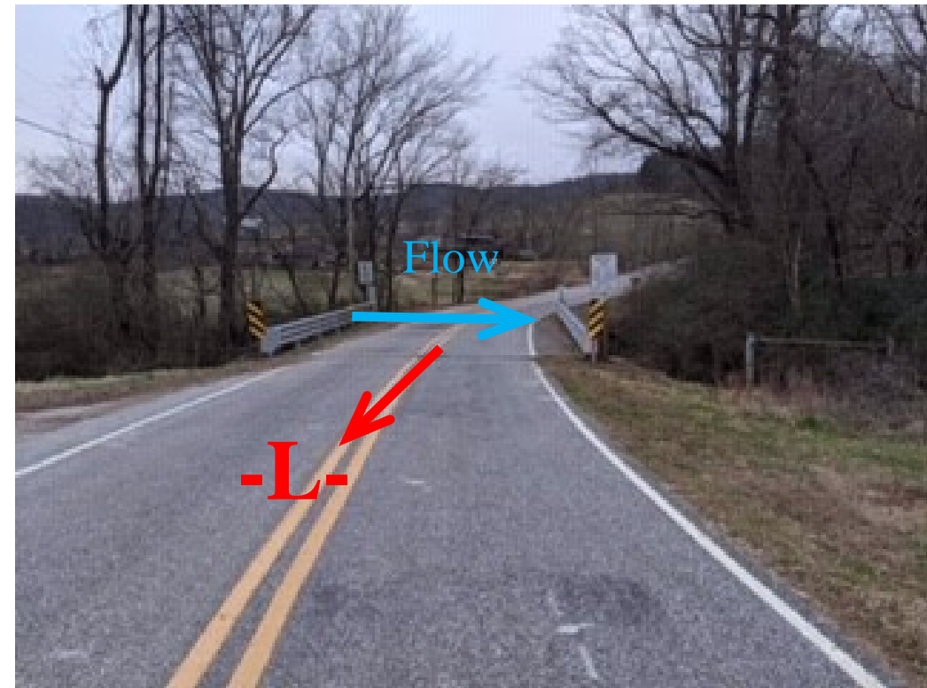
Looking South Toward End Bent 1
