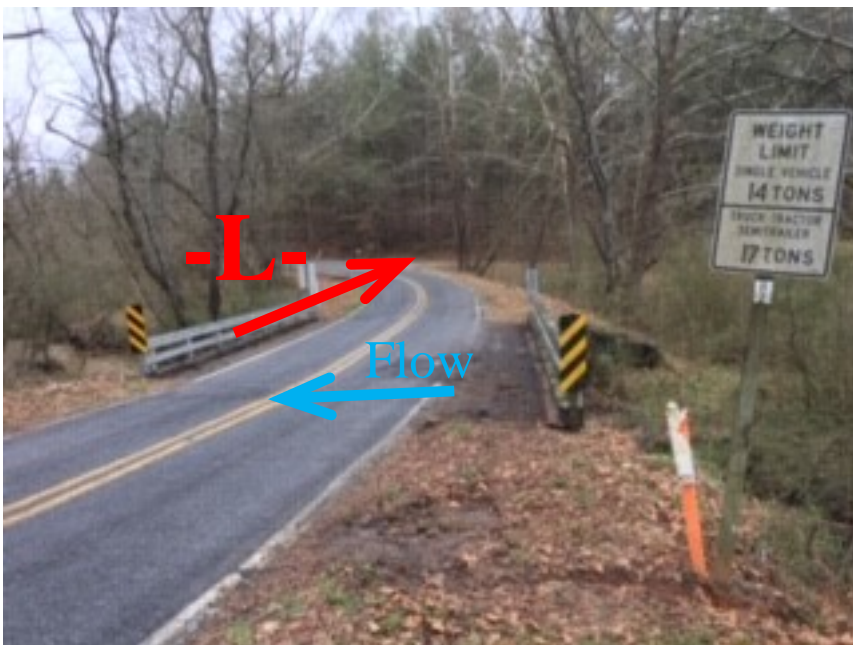
Looking South From End Bent 2
