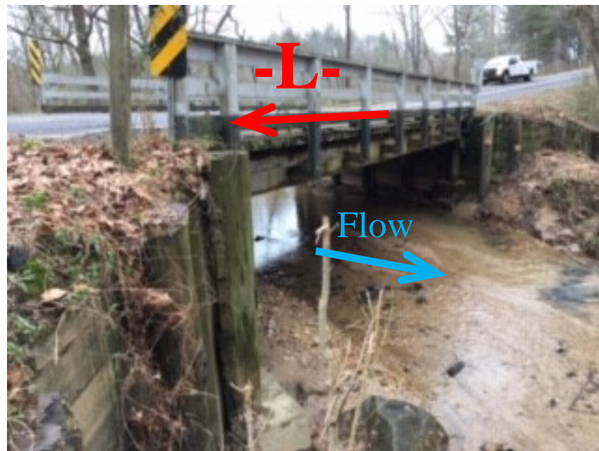
Looking South Toward End Bent 1
