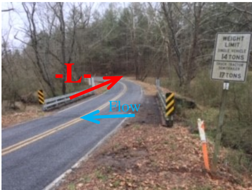
Looking South From End Bent 2
