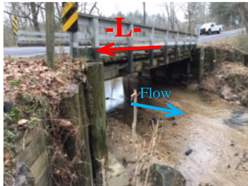
Looking South Toward End Bent 1
