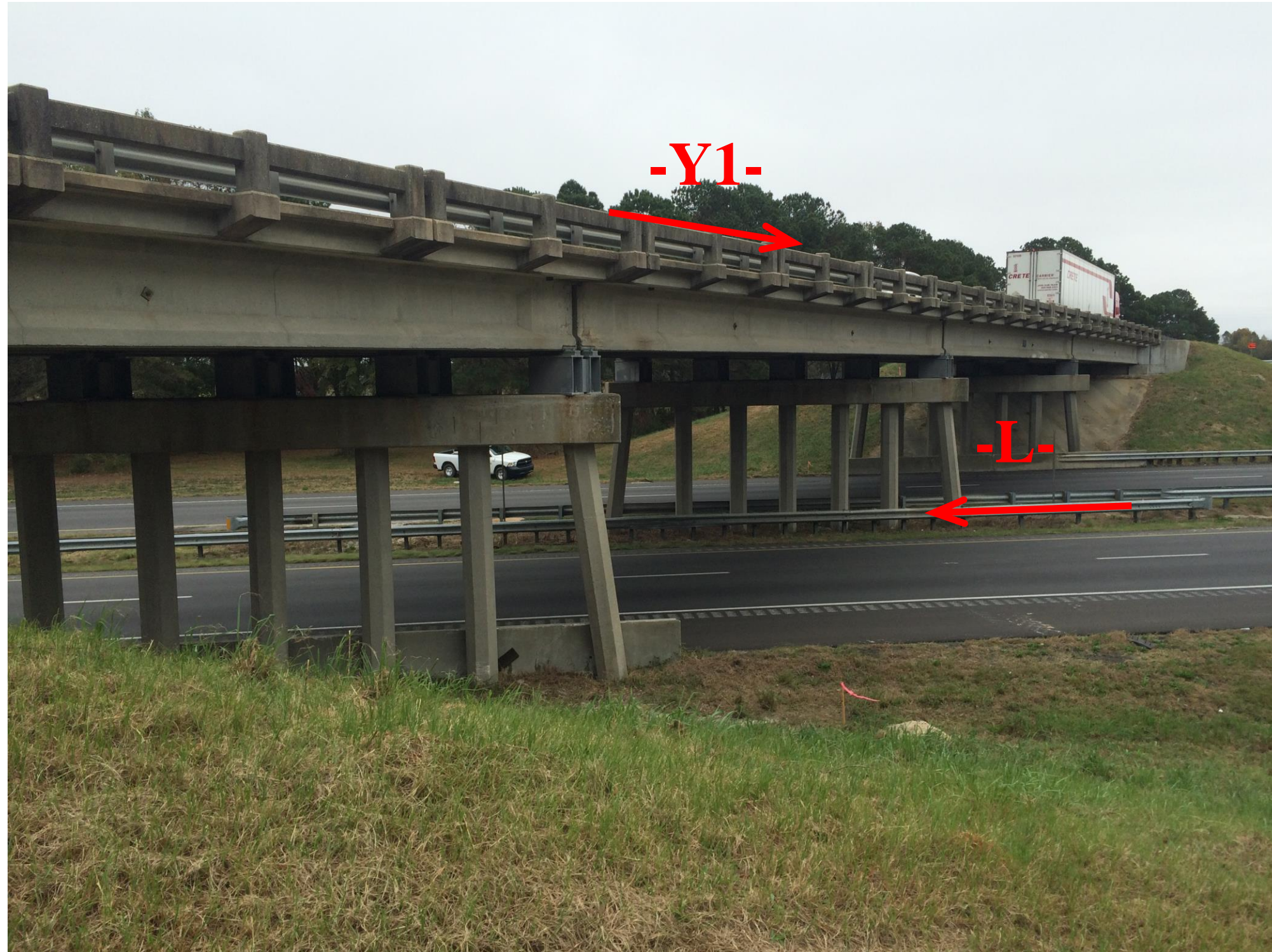
Looking Southeast towards End Bent 2
