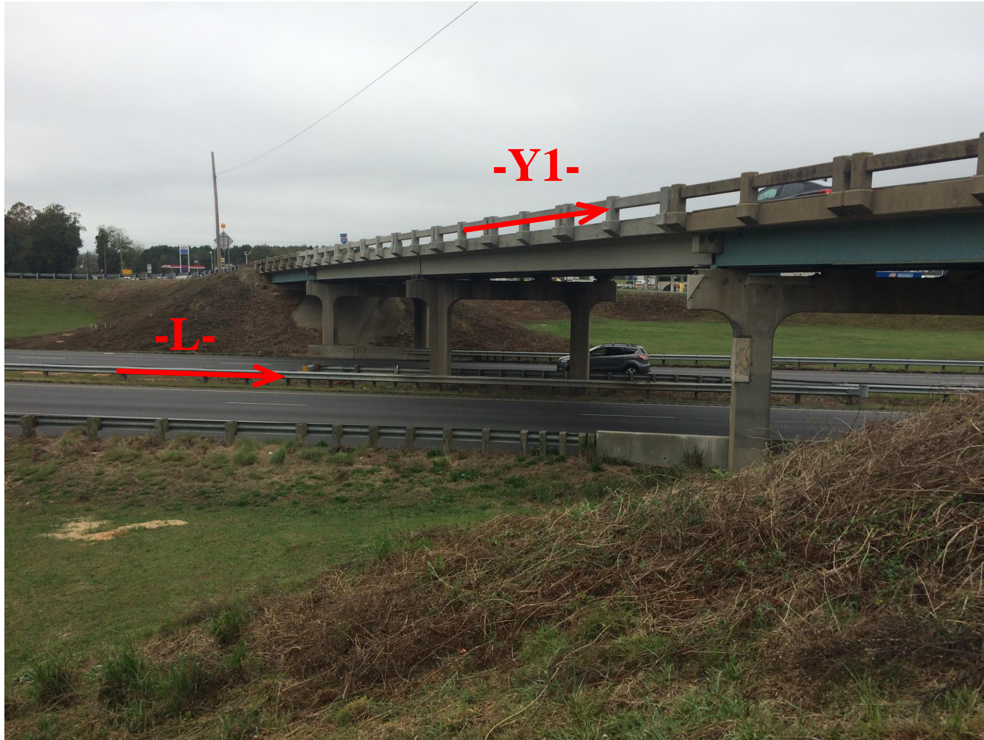
Looking West towards End Bent 1
