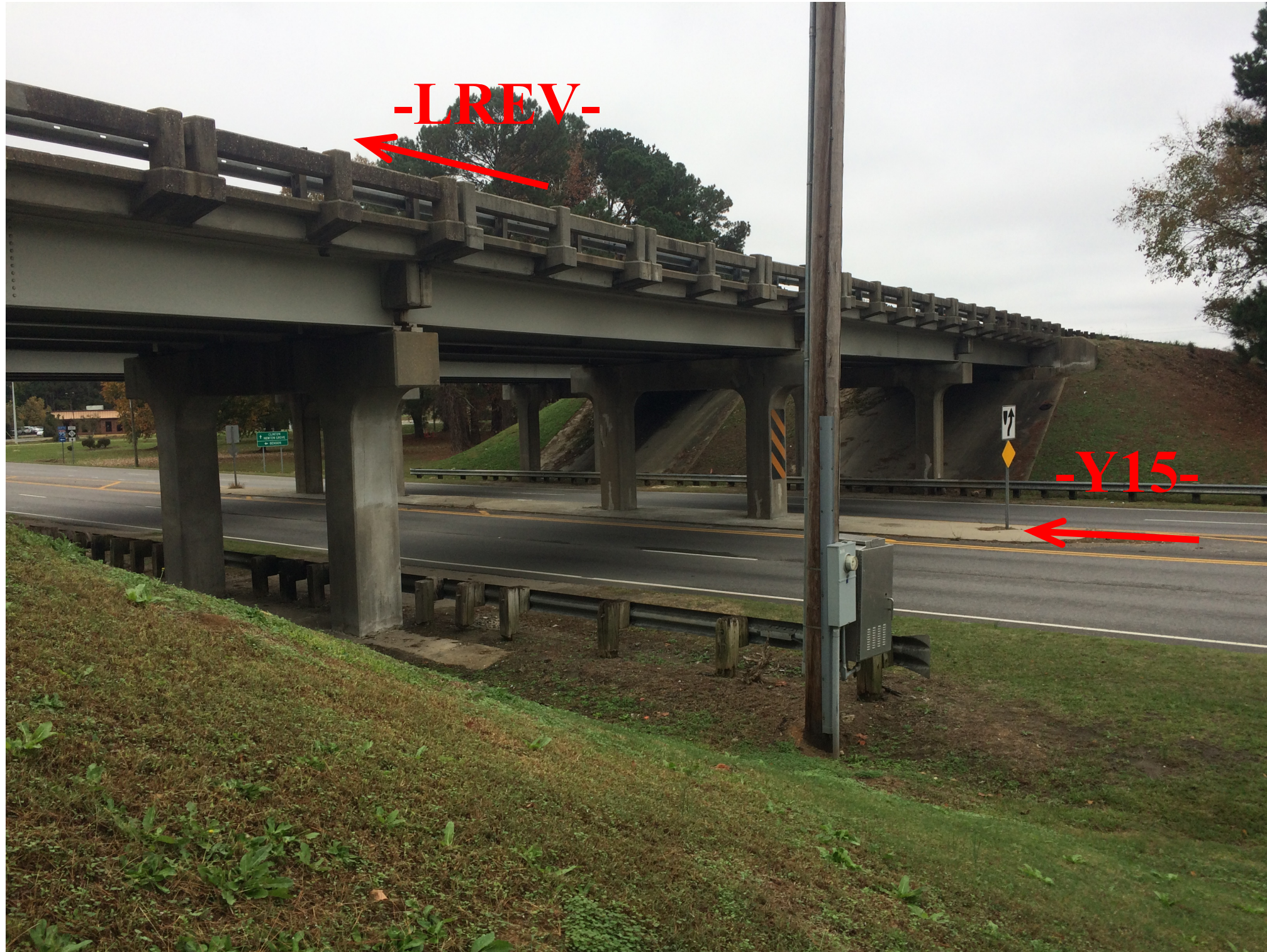
Looking South towards End Bent 1
