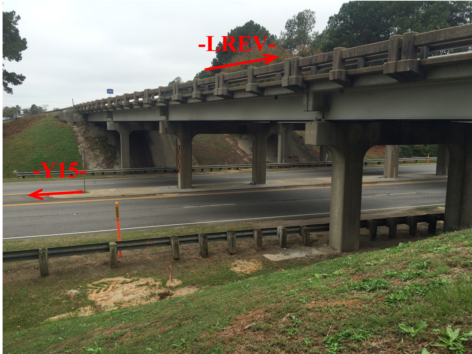
Looking Southwest towards End Bent 1
