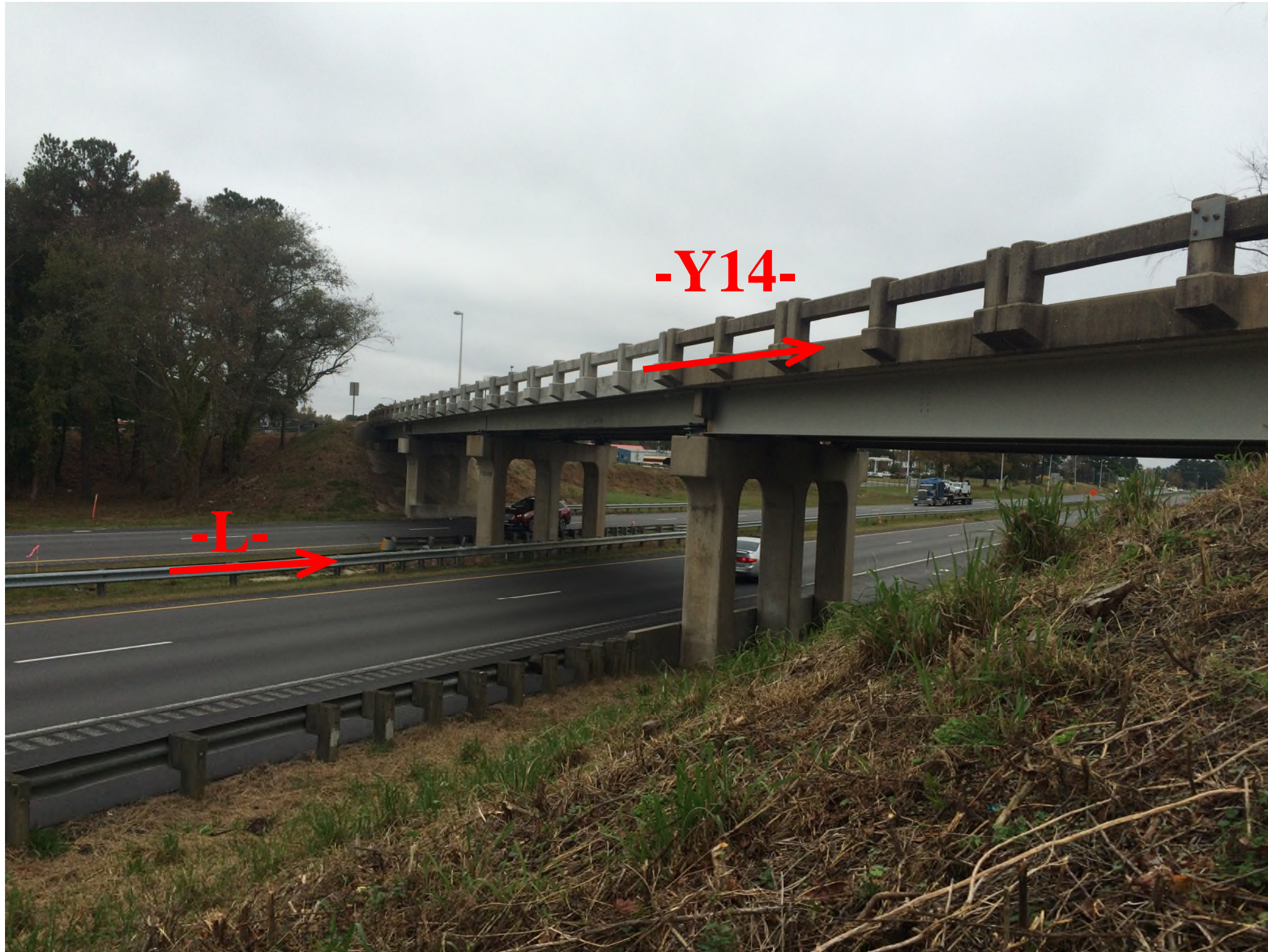
Looking West towards End Bent 1
