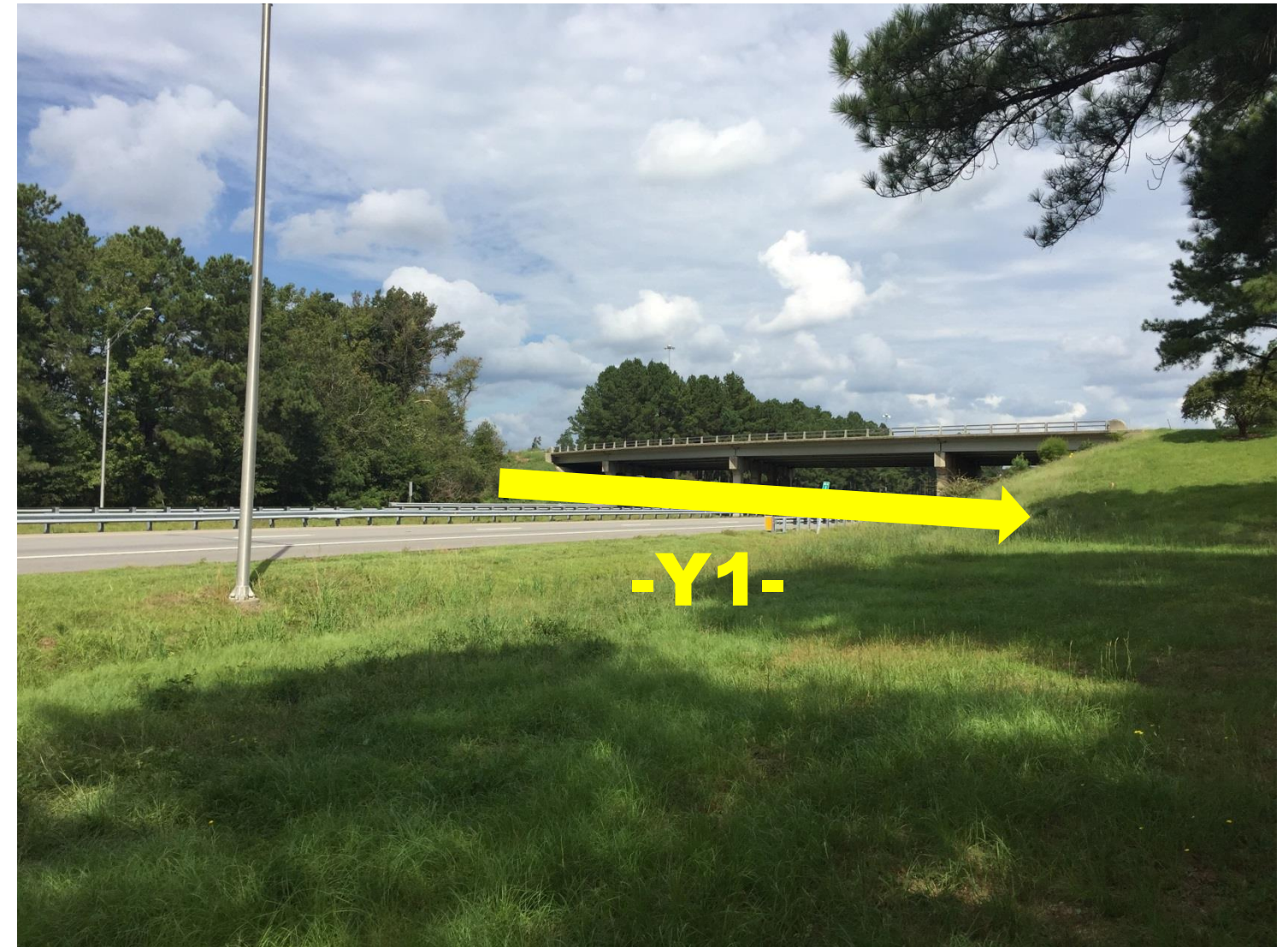
PHOTO TAKEN NEAR RPC-2000 LOOKING ALONG BRIDGE SPAN
