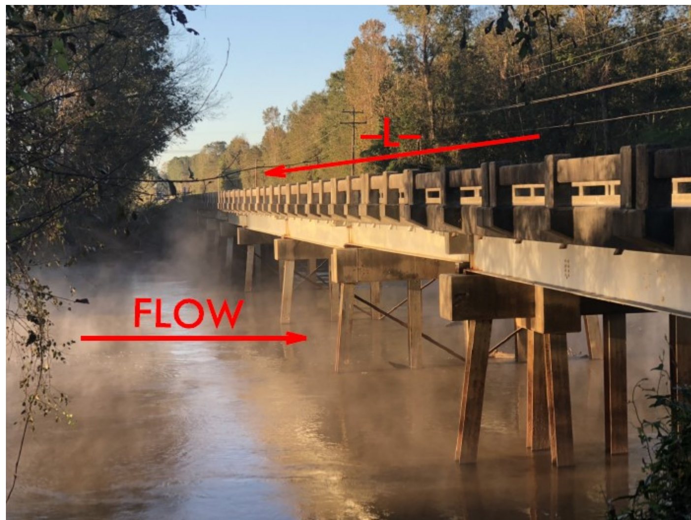
Looking North from End Bent 1
