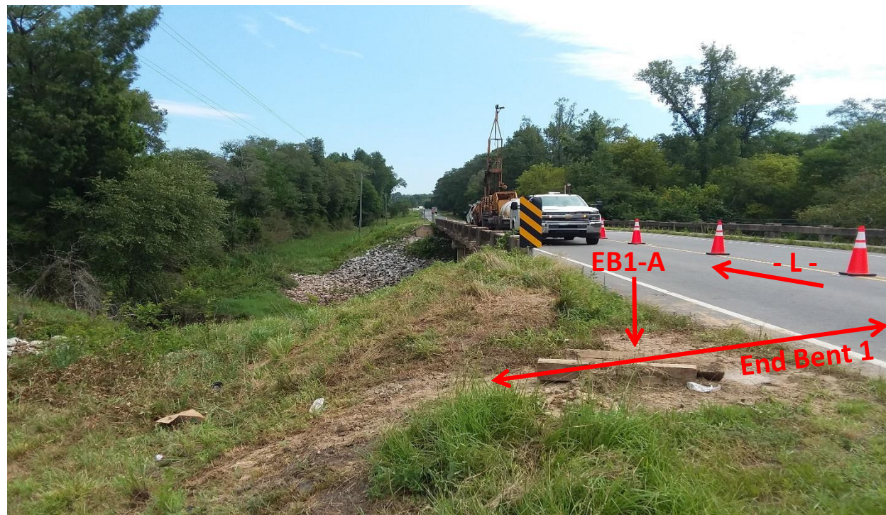
Photograph No. 2: View from End Bent 1 looking North
