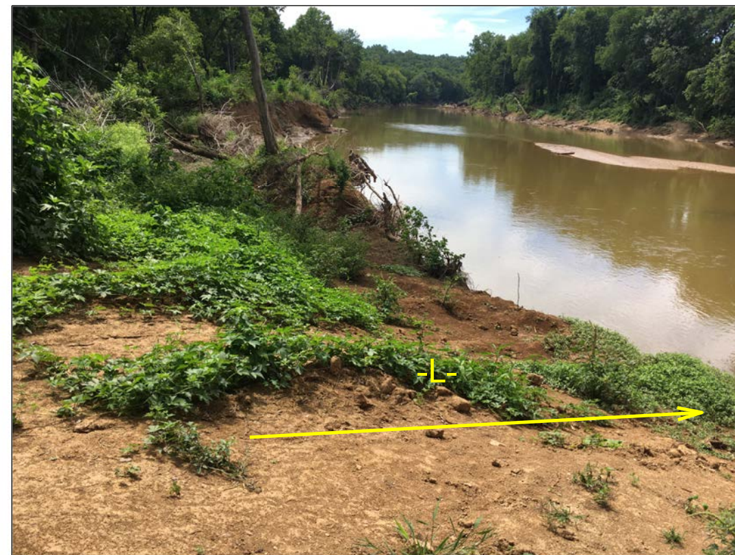
PHOTO 4: VIEW NEAR BENT 4, FACING EAST ALONG ROCKY RIVER.
