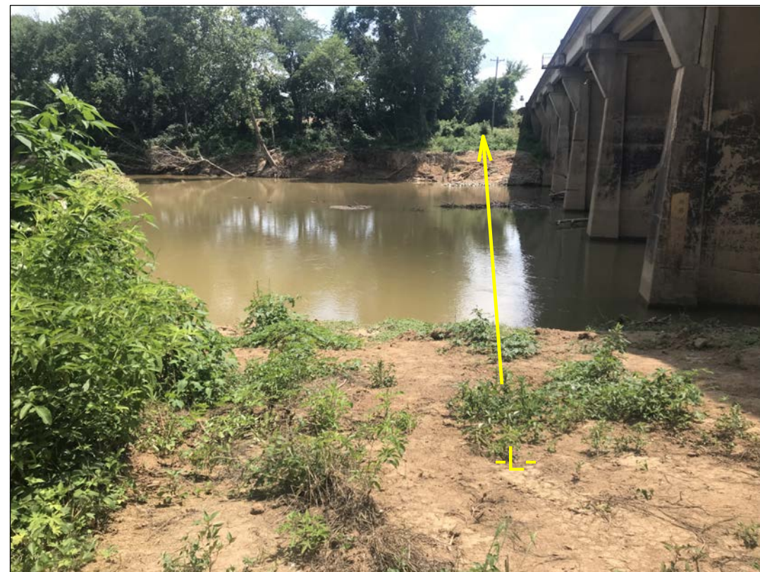
PHOTO 3: VIEW FROM BENT 4 FACING DOWNSTATION.
