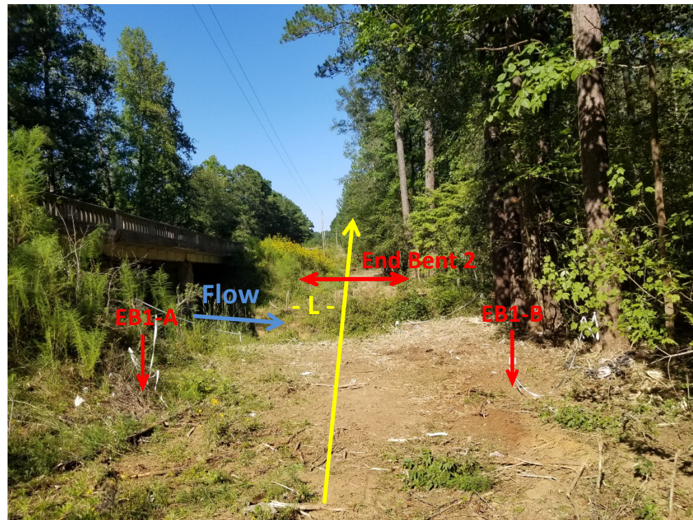
Photograph No. 1: View at End Bent 1 looking north
