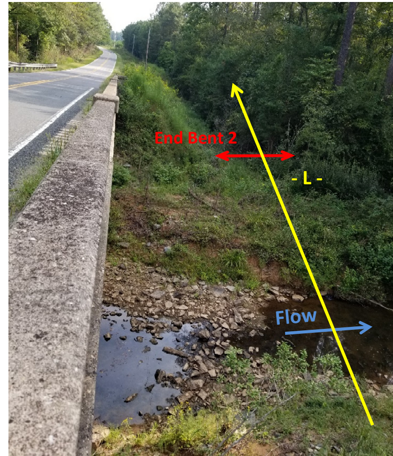
Photograph No. 3: View of End Bent 2 looking north
